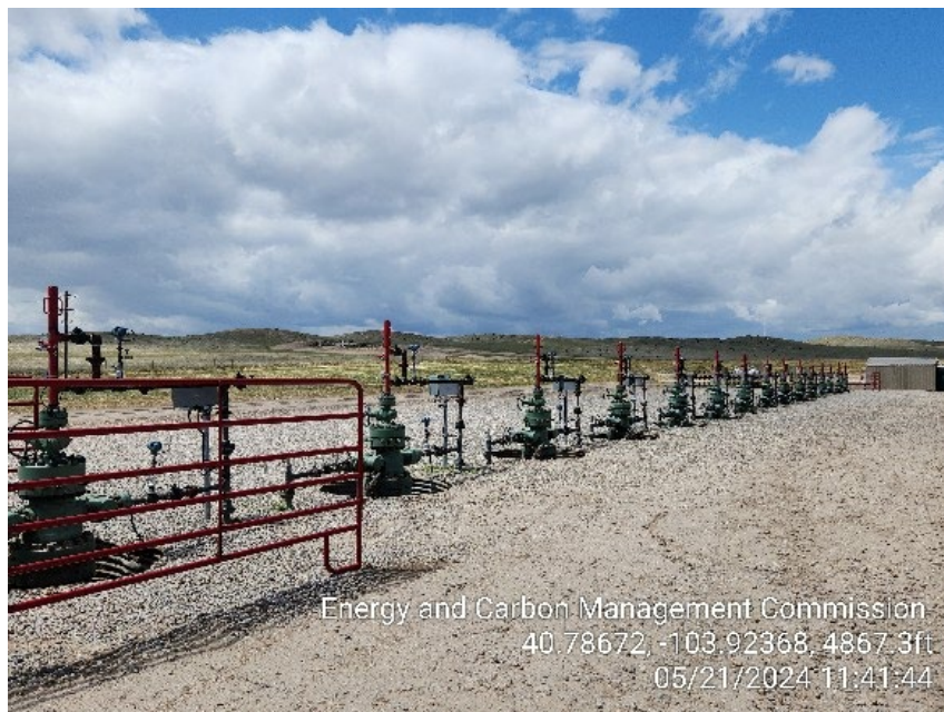
Photo 1 – Wellheads – Cellars not back filled in
