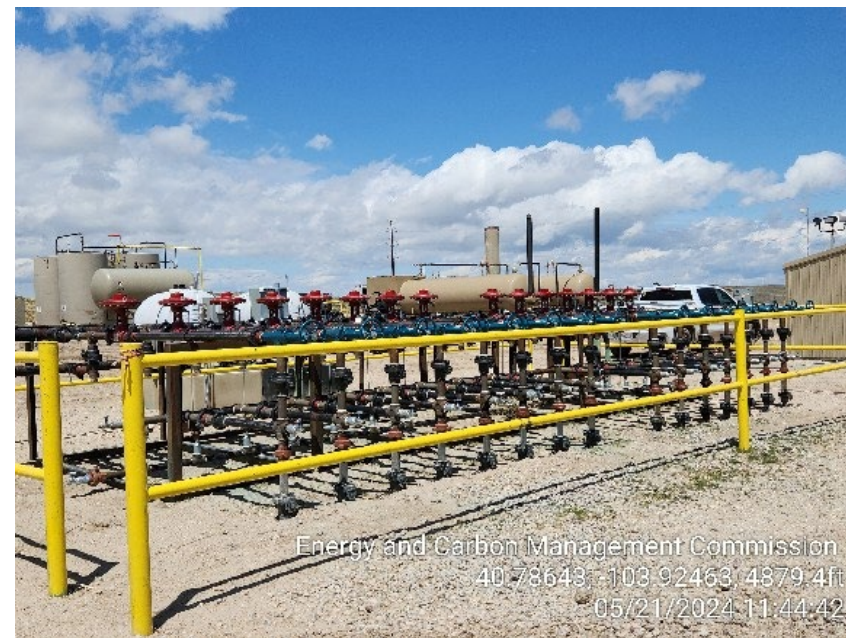
Photo 10 – Wellhead Headers
