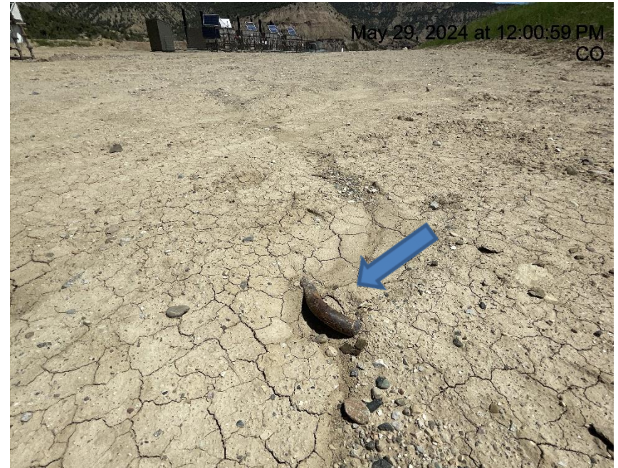
Photo # 8649 Same unmarked deadman from different angle
