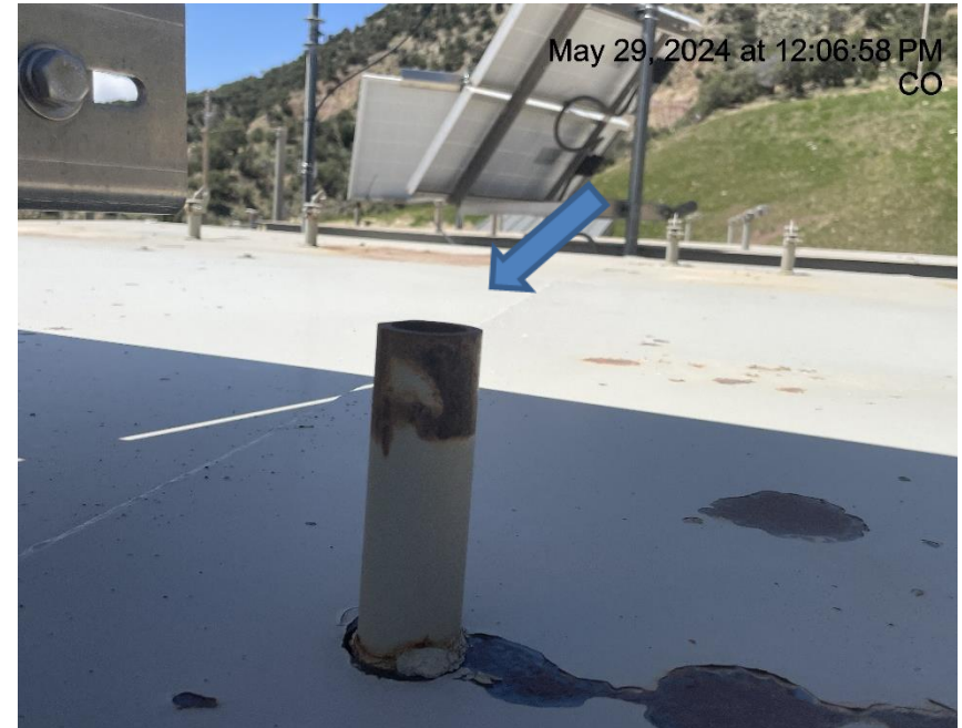
Photo # 8653 Rupture disc vent line does not comply with CECMC pressure safety device rules
