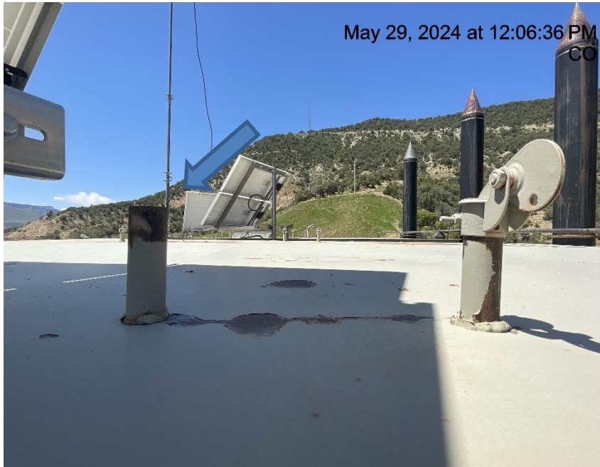
Photo # 8652 Rupture disc vent line does not comply with CECMC pressure safety device rules
