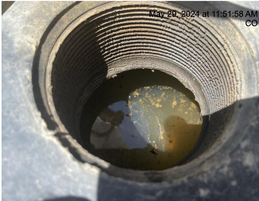
Photo # 8671 Failure to maintain chemical BMP/chemical containment full of fluid & not sufficient to contain possible spill
