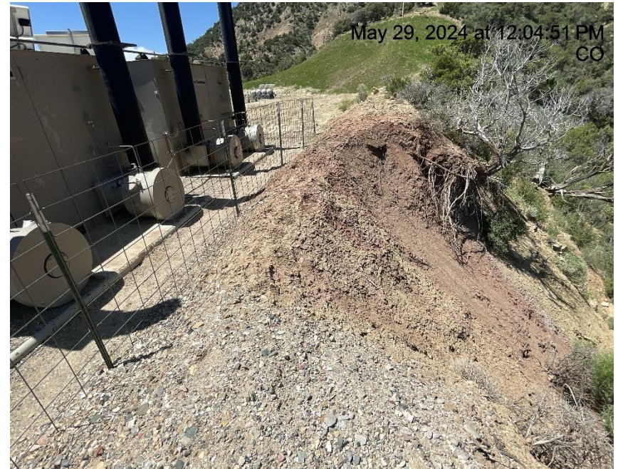
Photo # 8674 Edge of pad has started to slough & started to damage berm/BMP (N/NE area of pad behind production units)
