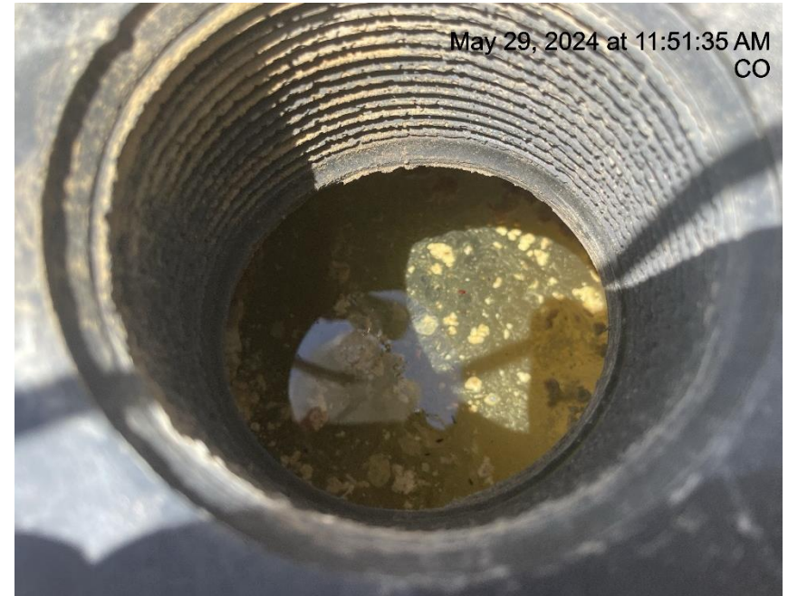
Photo # 8670 Failure to maintain chemical BMP/chemical containment full of fluid & not sufficient to contain possible spill
