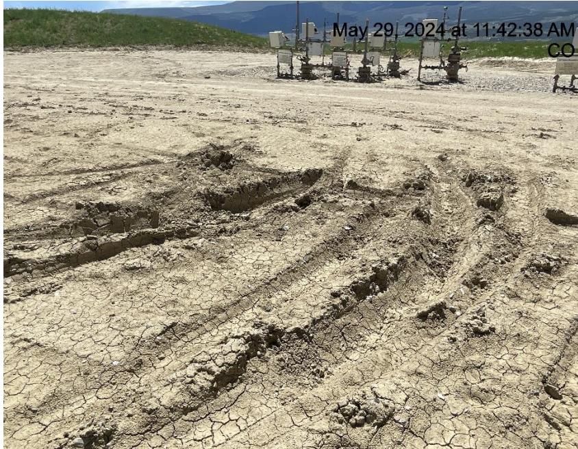
Photo # 8677 Lack of stabilization/compaction
