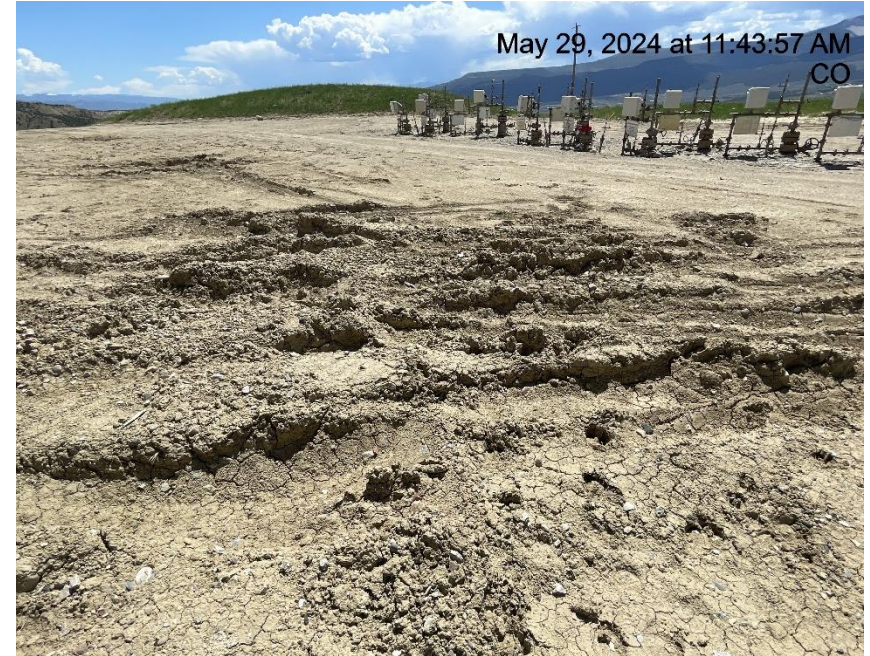
Photo # 8680 Lack of stabilization/compaction
