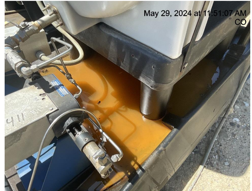
Photo # 8668 Failure to maintain chemical BMP/chemical containment full of fluid & not sufficient to contain possible spill
