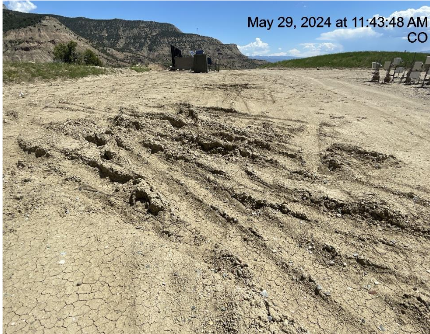
Photo # 8679 Lack of stabilization/compaction
