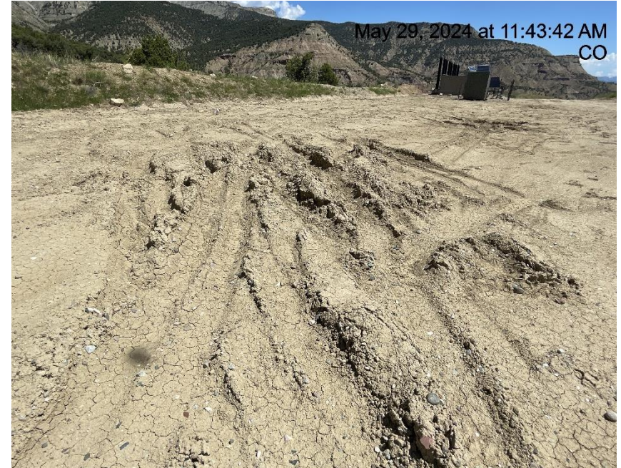
Photo # 8678 Lack of stabilization/compaction
