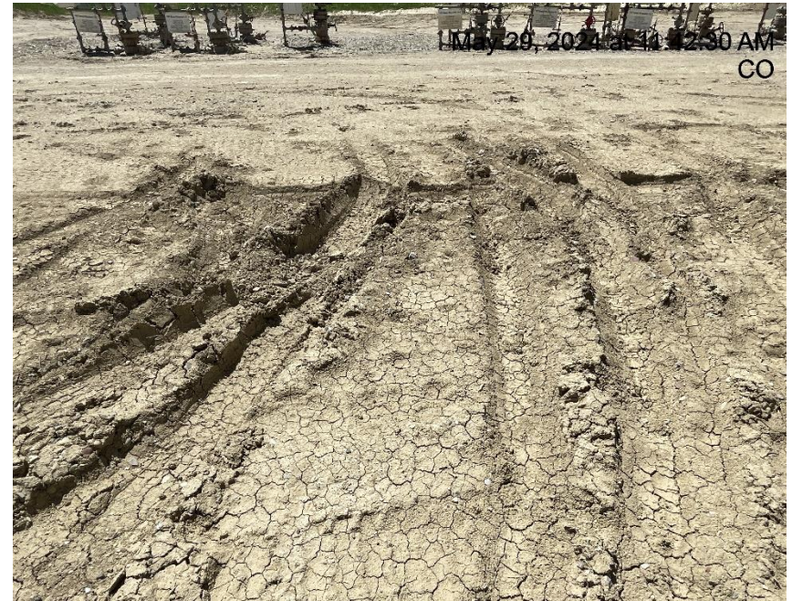
Photo # 8676 Lack of stabilization/compaction
