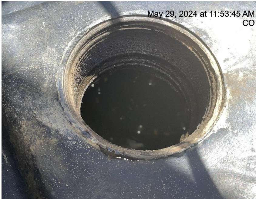
Photo # 8673 Failure to maintain chemical BMP/chemical containment 7/8 th full of fluid & not sufficient to contain possible spill
