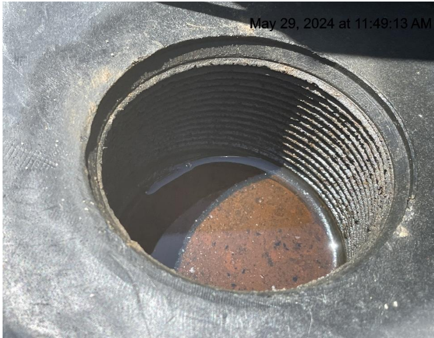
Photo # 8669 Failure to maintain chemical BMP/chemical containment full of fluid & not sufficient to contain possible spill
