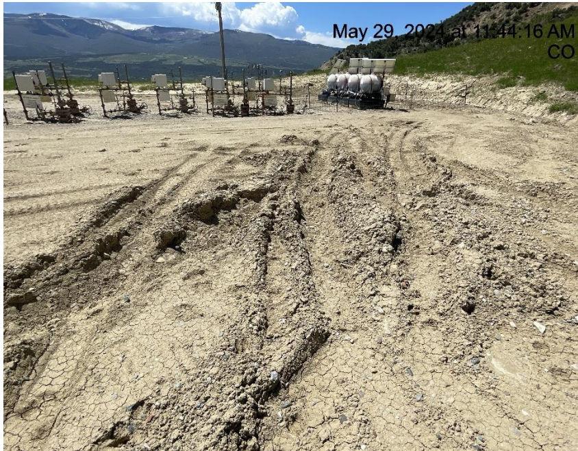
Photo # 8681 Lack of stabilization/compaction
