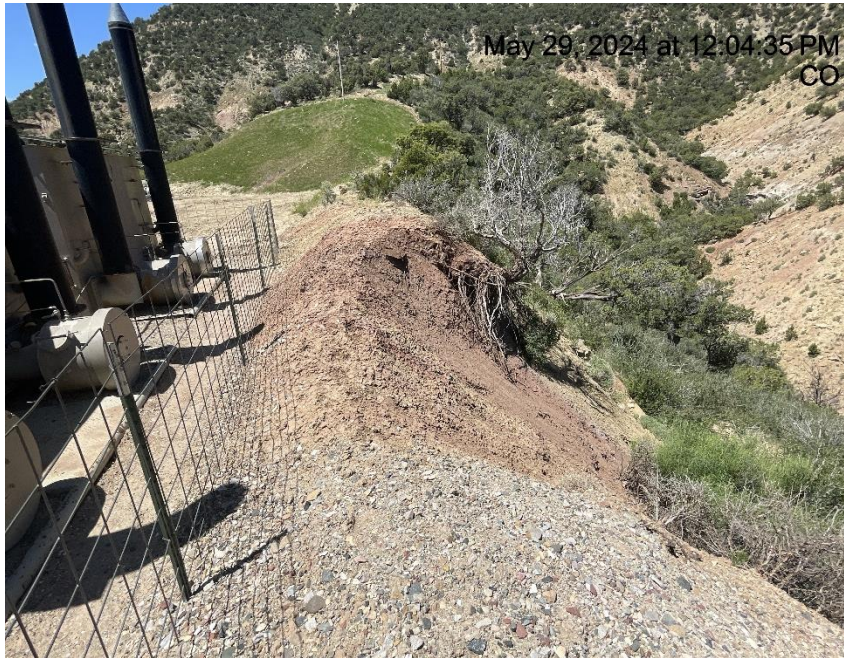
Photo # 8675 Edge of pad has started to slough & started to damage berm/BMP (N/NE area of pad behind production units)
