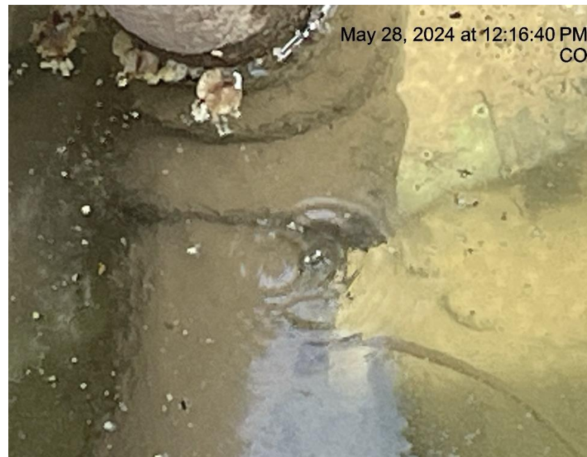
Photo # 8476 Possible leak/gas bubbling up through water in cellar around bradenhead line
