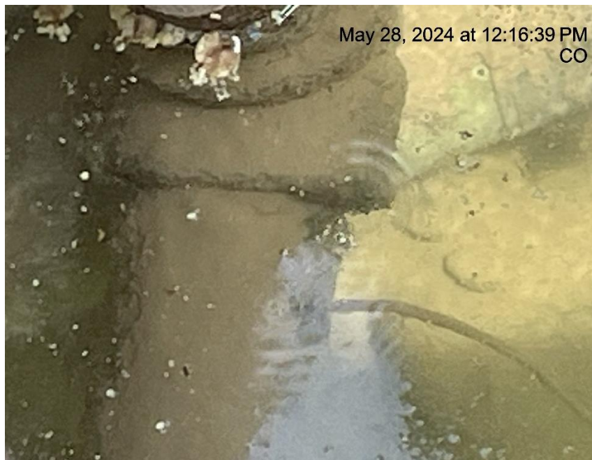
Photo # 8475 Possible leak/gas bubbling up through water in cellar around bradenhead line
