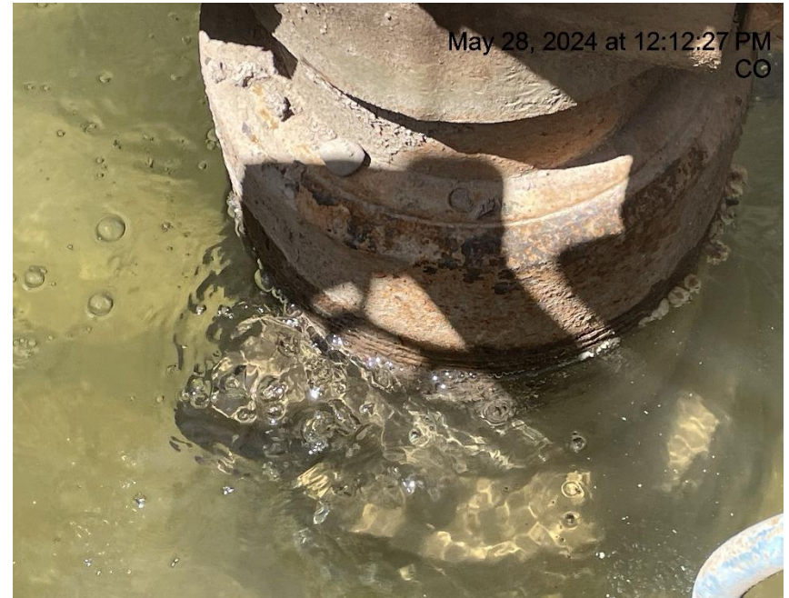
Photo # 8472 Possible wellhead leak/gas bubbling up around wellhead through water in cellar
