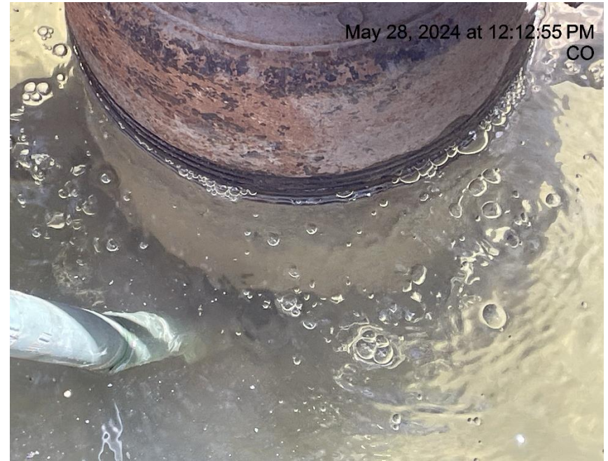
Photo # 8474 Possible wellhead leak/gas bubbling up around wellhead through water in cellar
