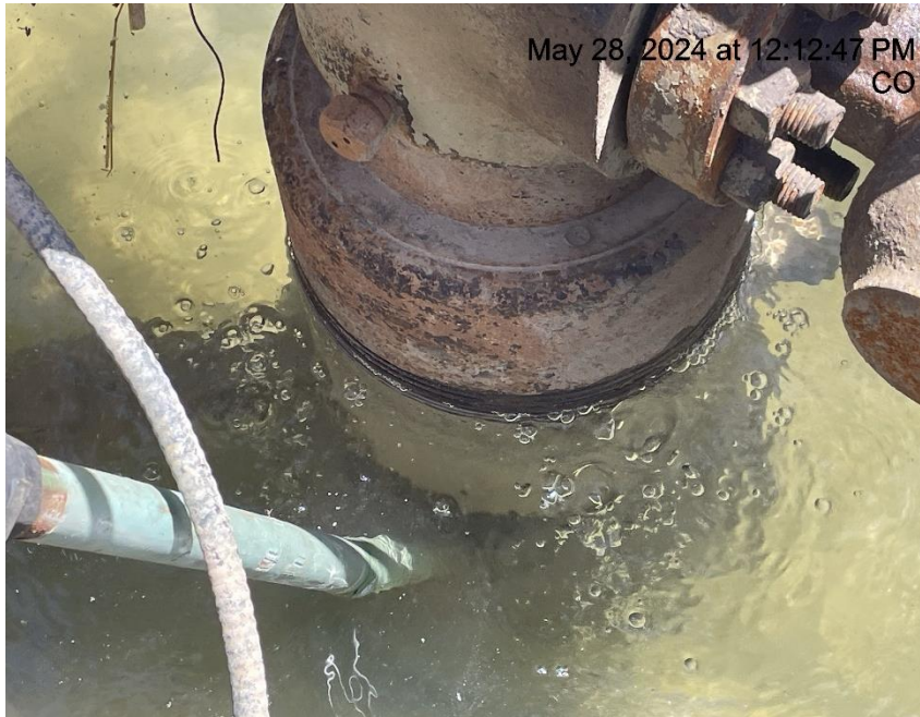
Photo # 8473 Possible wellhead leak/gas bubbling up around wellhead through water in cellar
