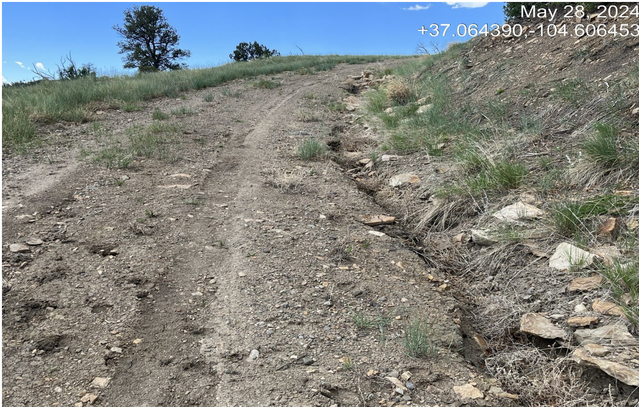
Photo 2. Facing southwest. There is an erosion along this area which should be repaired with BMP's
