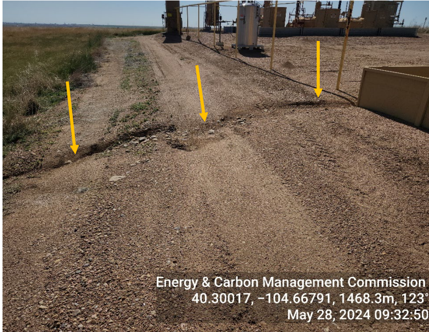
Photo 7: Erosion NE of tank battery berm
