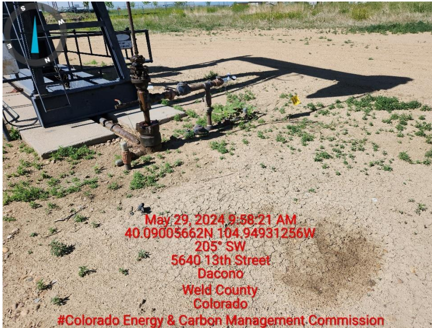
Photo 5 stained soil around well and in front of well
