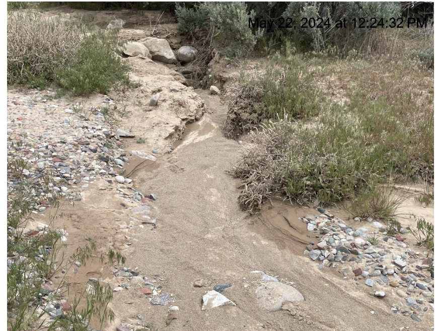
Photo # 7894 Erosion & transport of sediment onto lease road
