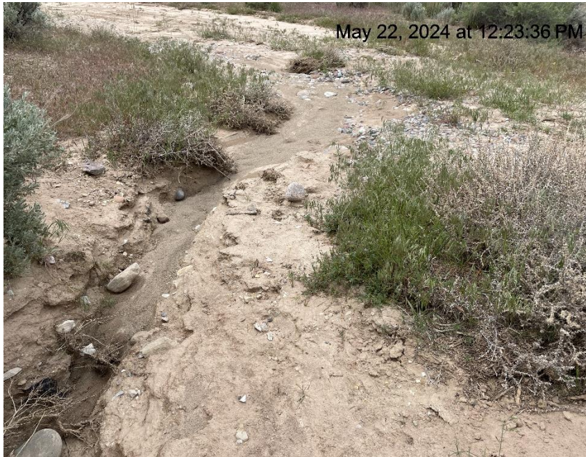
Photo # 7893 Erosion & transport of sediment onto lease road
