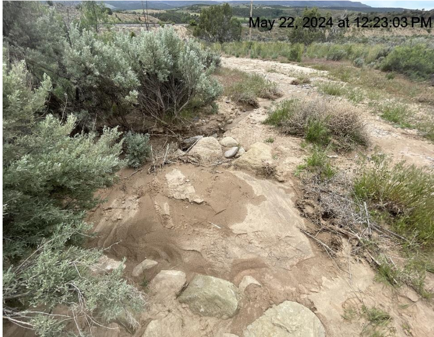
Photo # 7891 Ditch & Culvert need maintenance/erosion & transport of sediment onto lease road
