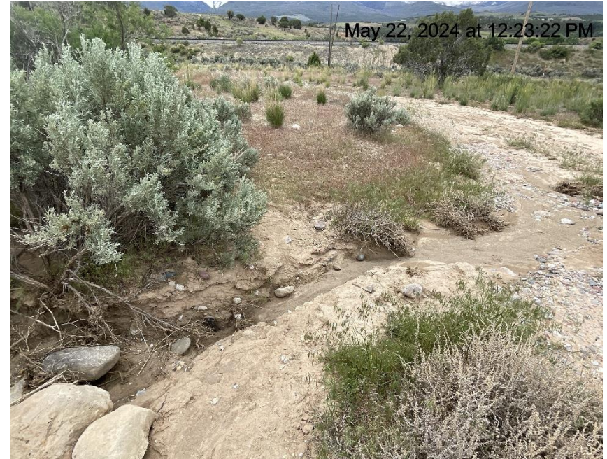
Photo # 7892 Erosion & transport of sediment onto lease road
