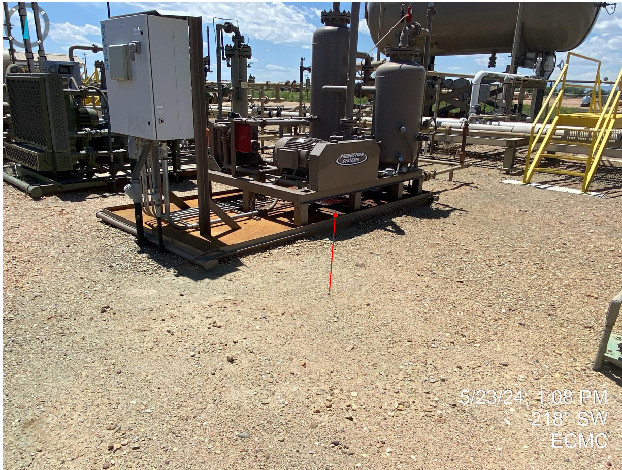
Photo 30. Free fluids observed on skid need to be properly disposed of per Rule 905.e.
