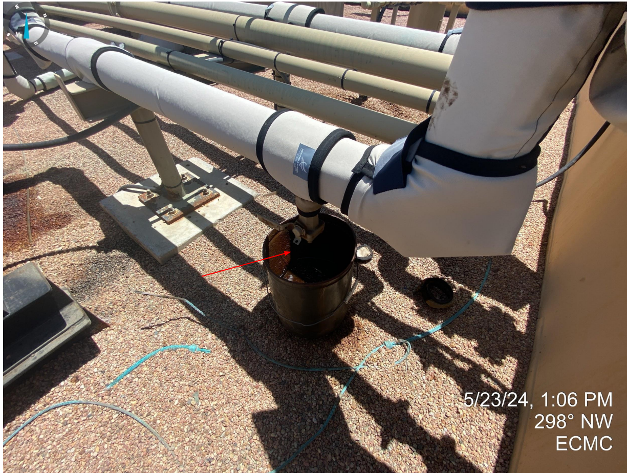
Photo 24. No wildlife protection equipment observed on bucket.
