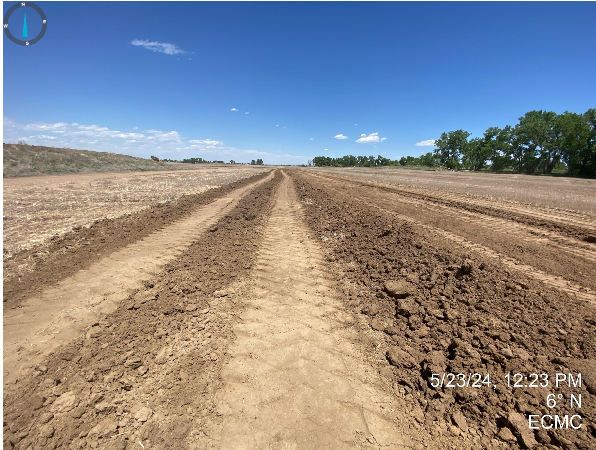
Photo 7. East side of pad expansion. It appears that the existing topsoil stockpile is being moved further east to the new DA limits. Operator shall ensure that all topsoil is salvaged in accordance with Rule 1002.b and that topsoil is not used as fill material.
