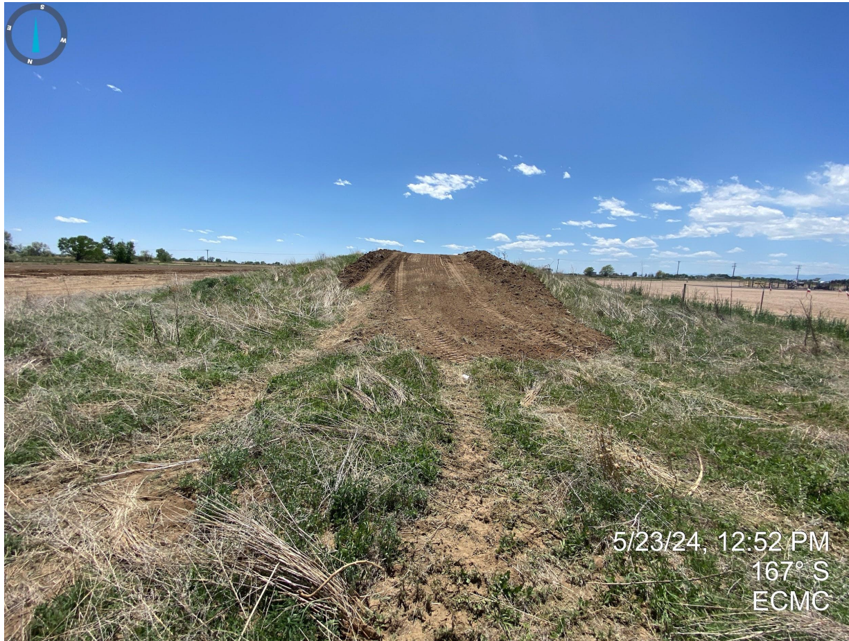
Photo 13. North side of existing topsoil stockpile. It appears that topsoil is in the process of being moved further east due to pad expansion. CO List C Noxious Weed (field bindweed and downy brome) are the predominant vegetation cover on the topsoil stockpile at the time of this inspection.
