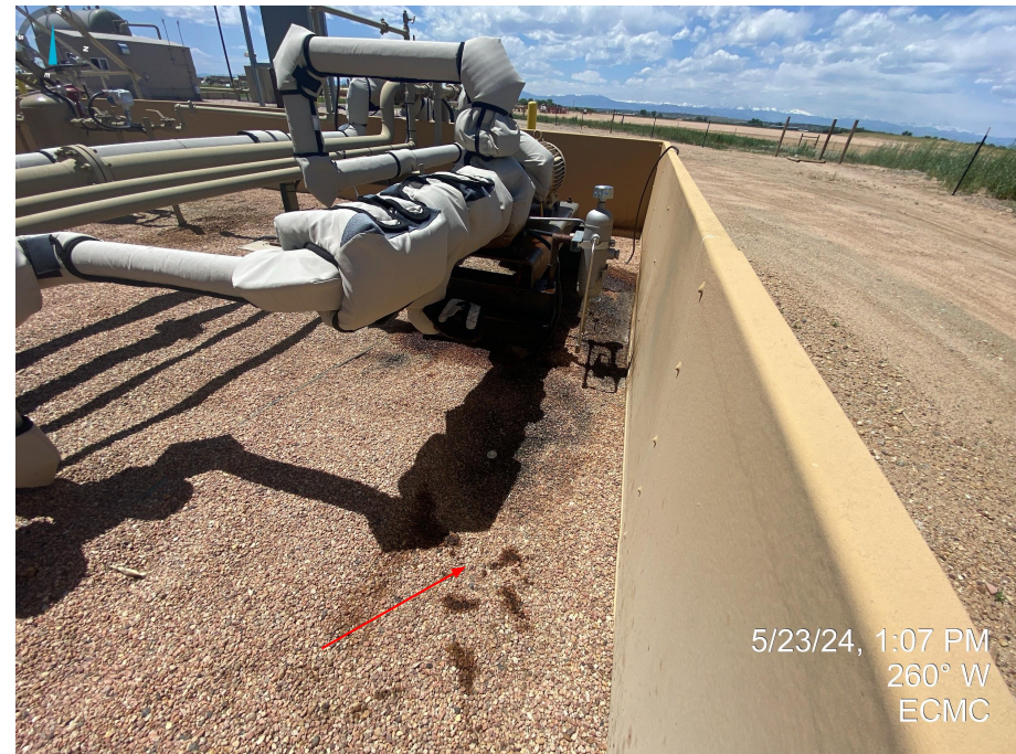
Photos 22 & 23. Stained soils observed near equipment in tank battery secondary containment.
