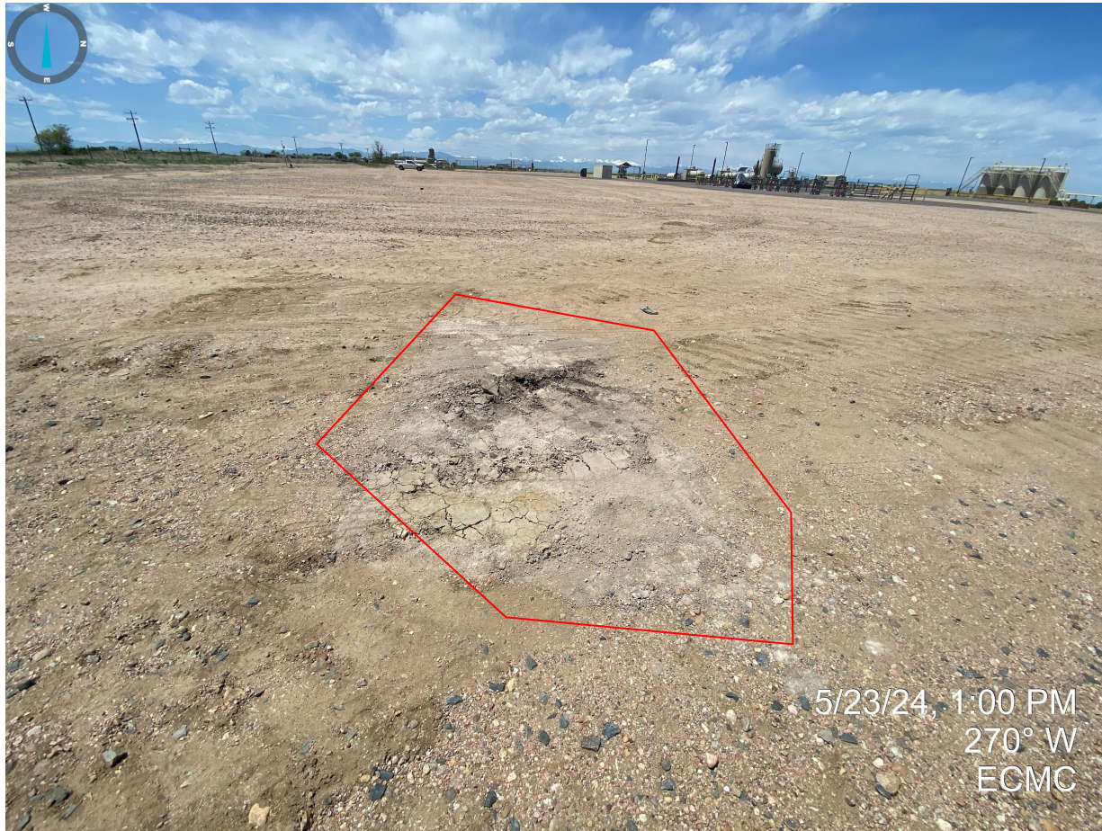
Photo 18. Unmix concrete debris is a potential stormwater pollutant source and needs to be removed and disposed of.
