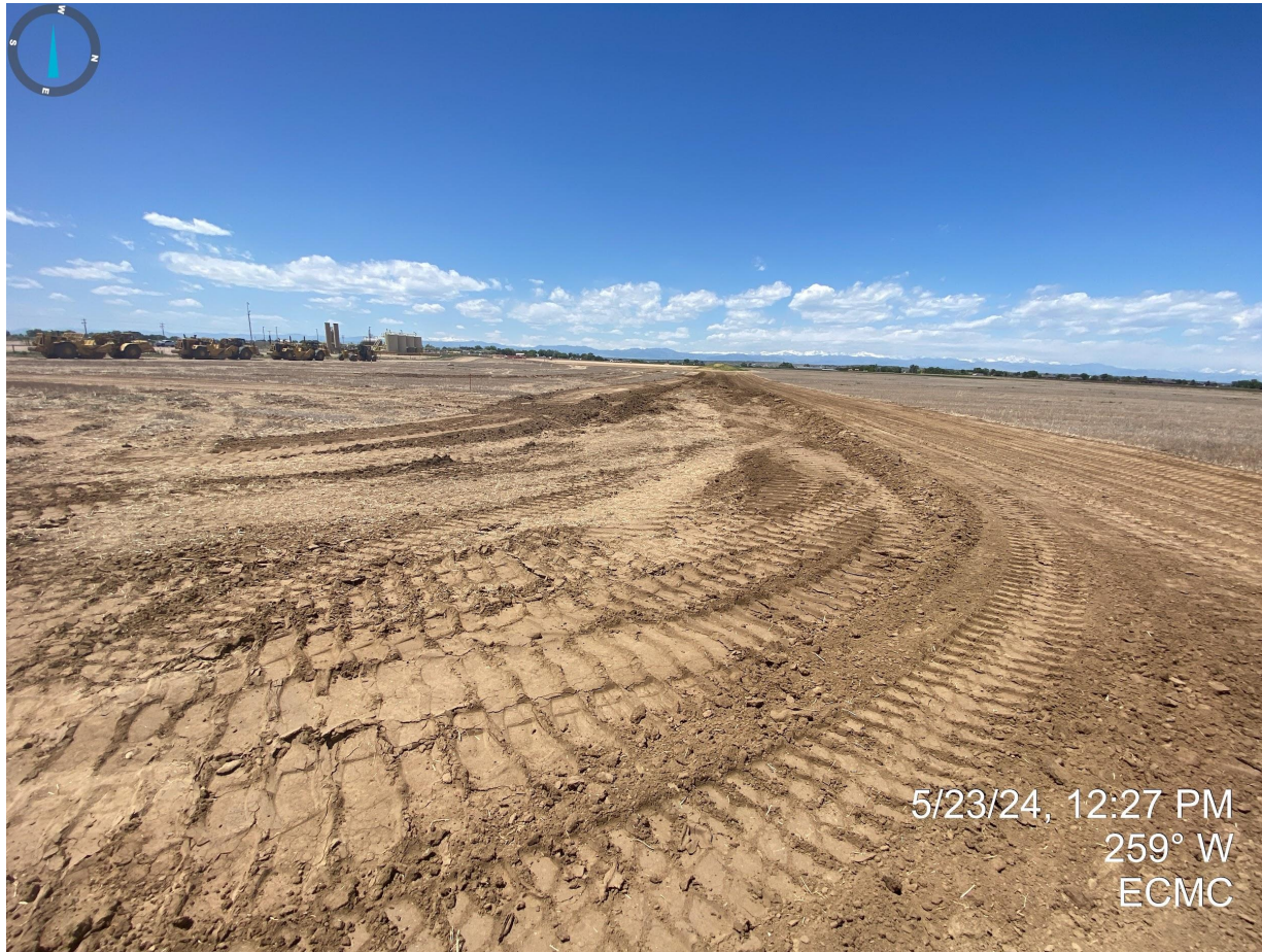
Photo 8. Northeast corner of pad expansion. Perimeter stormwater controls are still in process at the time of this inspection.
