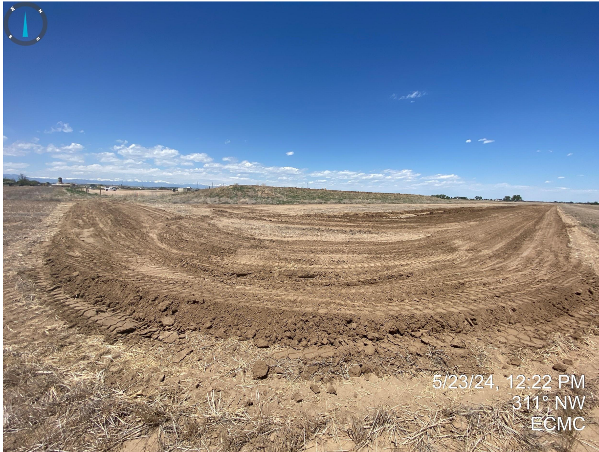
Photo 6. Southeast corner of pad expansion. Perimeter stormwater controls are still in process at the time of this inspection.
