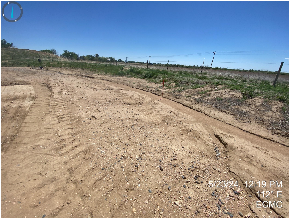
Photo 3. Southeast corner of the production area near the sediment trap. Erosion degradation observed at the time of this inspection.
