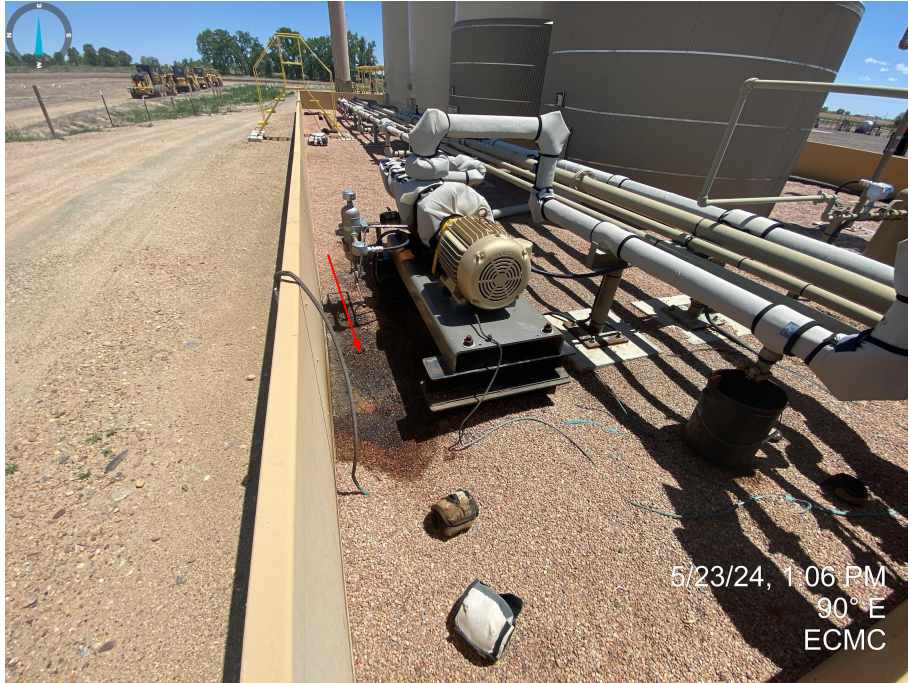
Photos 22 & 23. Stained soils observed near equipment in tank battery secondary containment.
