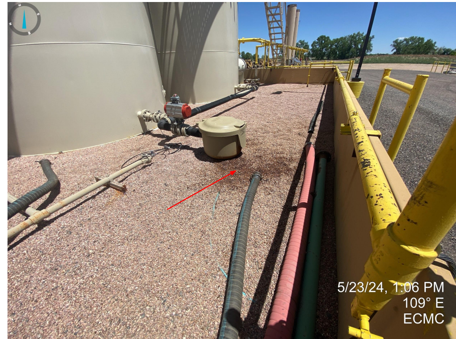
Photos 20 & 21. Stained soil observed within secondary containment at tank battery.
