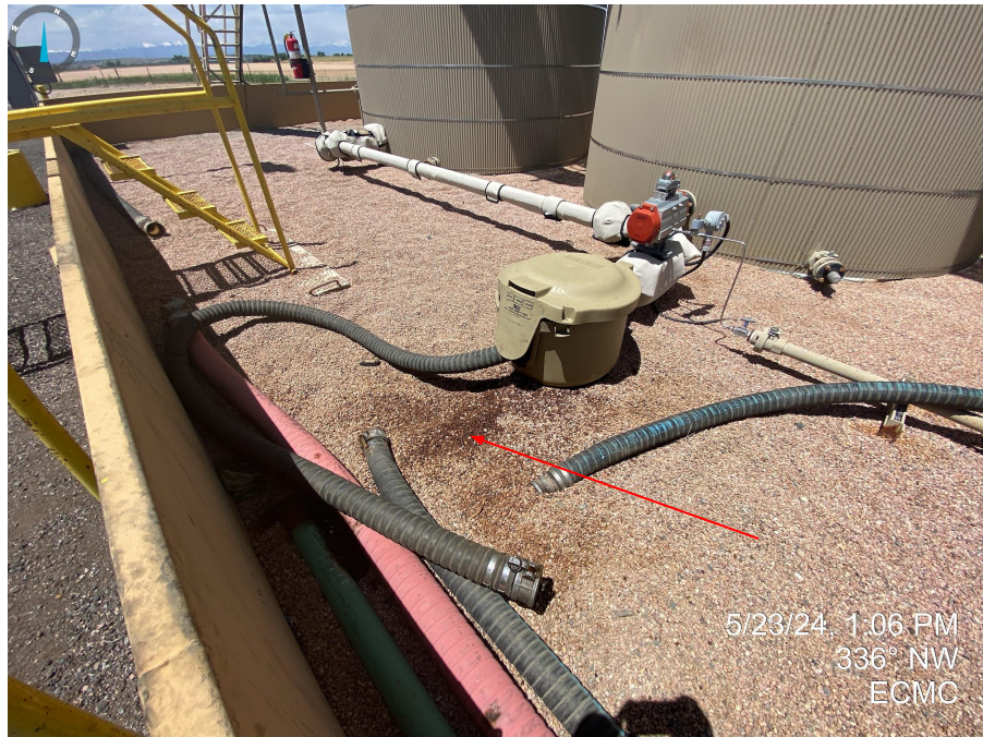
Photos 20 & 21. Stained soil observed within secondary containment at tank battery.
