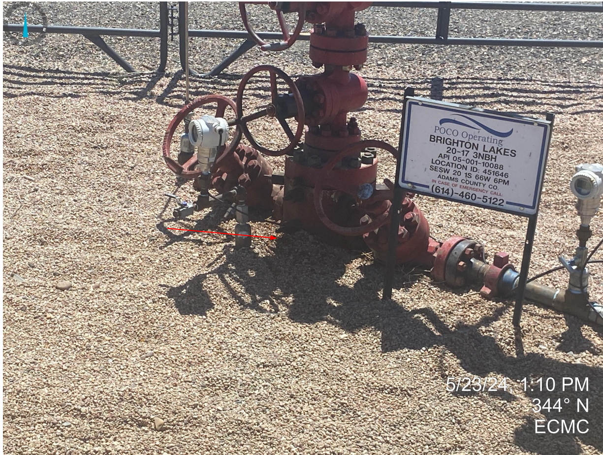
Photo 35. Stained soil observed near wellhead need to be properly disposed of per Rule 905.e.
