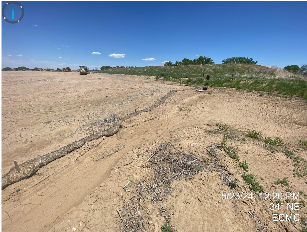
Photo 5. Sediment trap at the southeast corner of the location. Evidence of erosion degradation and inadequate BMPs (straw wattles).
