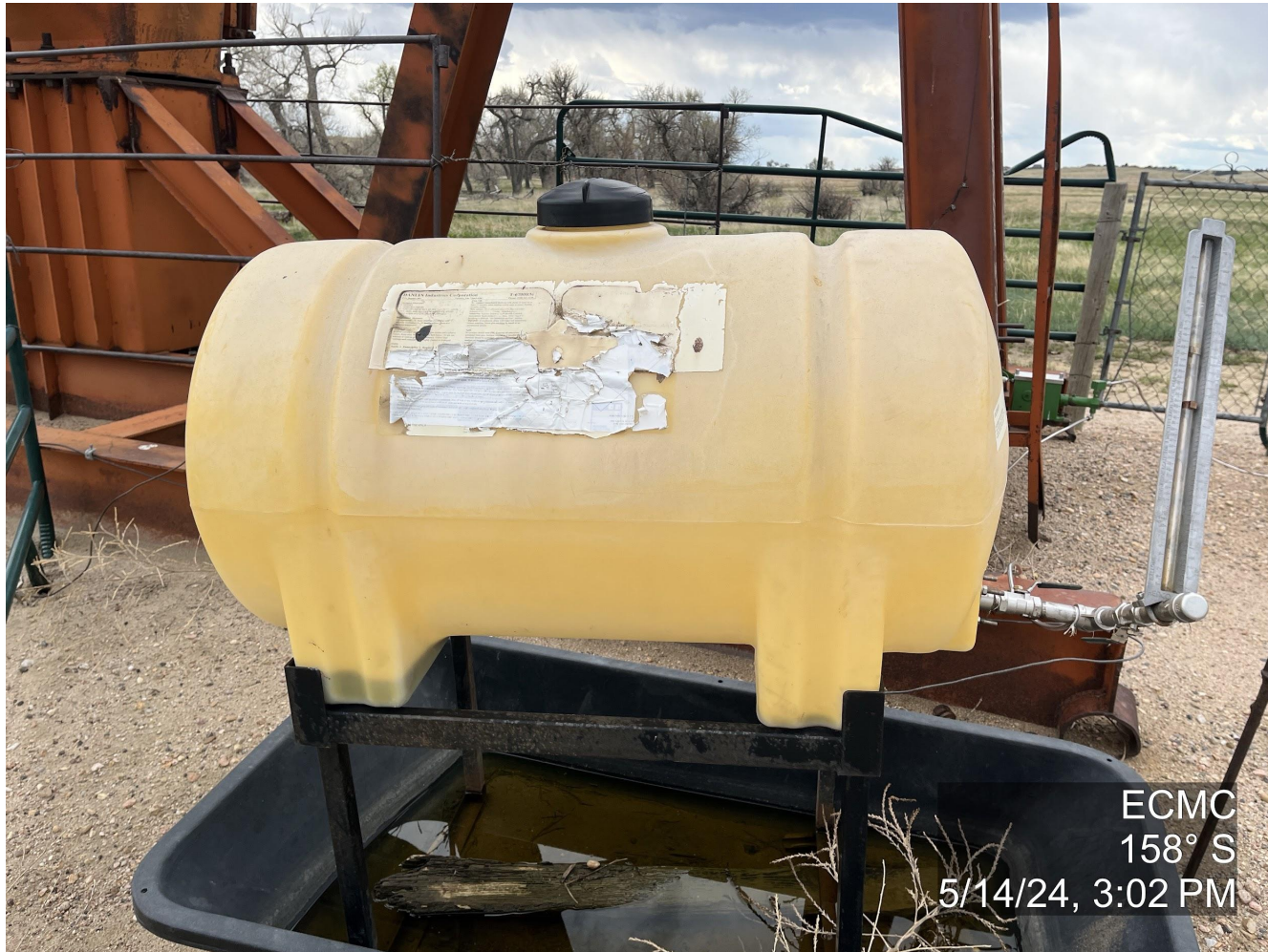
Photo 11. The photo was taken at the well location facing South. The photo illustrates tank placards need replacing and secondary containment is missing wildlife netting.
