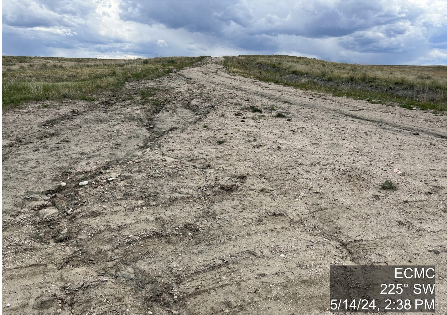
Photo 12. The photo was taken at the tank battery location facing Southwest. The photo illustrates the erosion for both the well and tank battery locations begins above the location on the access road and should be treated from top to bottom.
