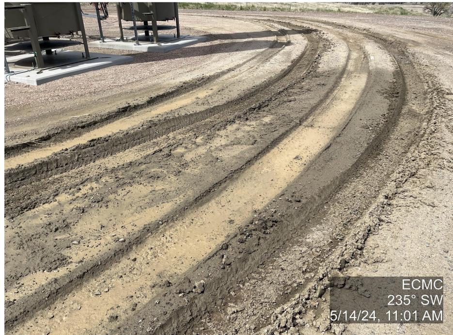
**Photo 6.** The photo was taken at the well location facing Southwest. The photo illustrates vehicle tracking through water ponding on the production pad.
