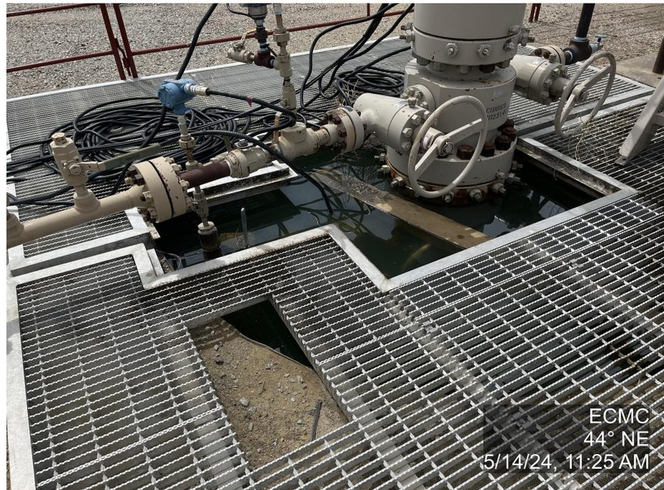
**Photo 8.** The photo was taken at the well location facing Northeast. The photo illustrates the grate around the wellhead is not sufficient to keep out wildlife and the cellar is full of water which has floated the wooden wildlife ramp that also appears to not be sufficient as a wildlife BMP.
