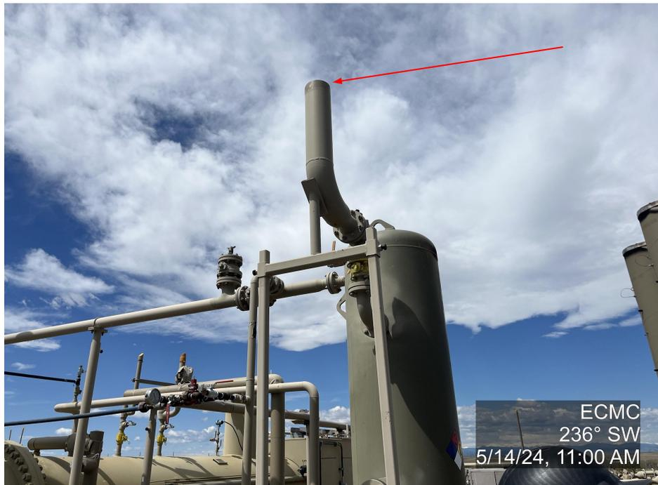
**Photo 5.** The photo was taken at the well location facing Southwest. The photo illustrates a missing cover on the exhaust of production equipment.
