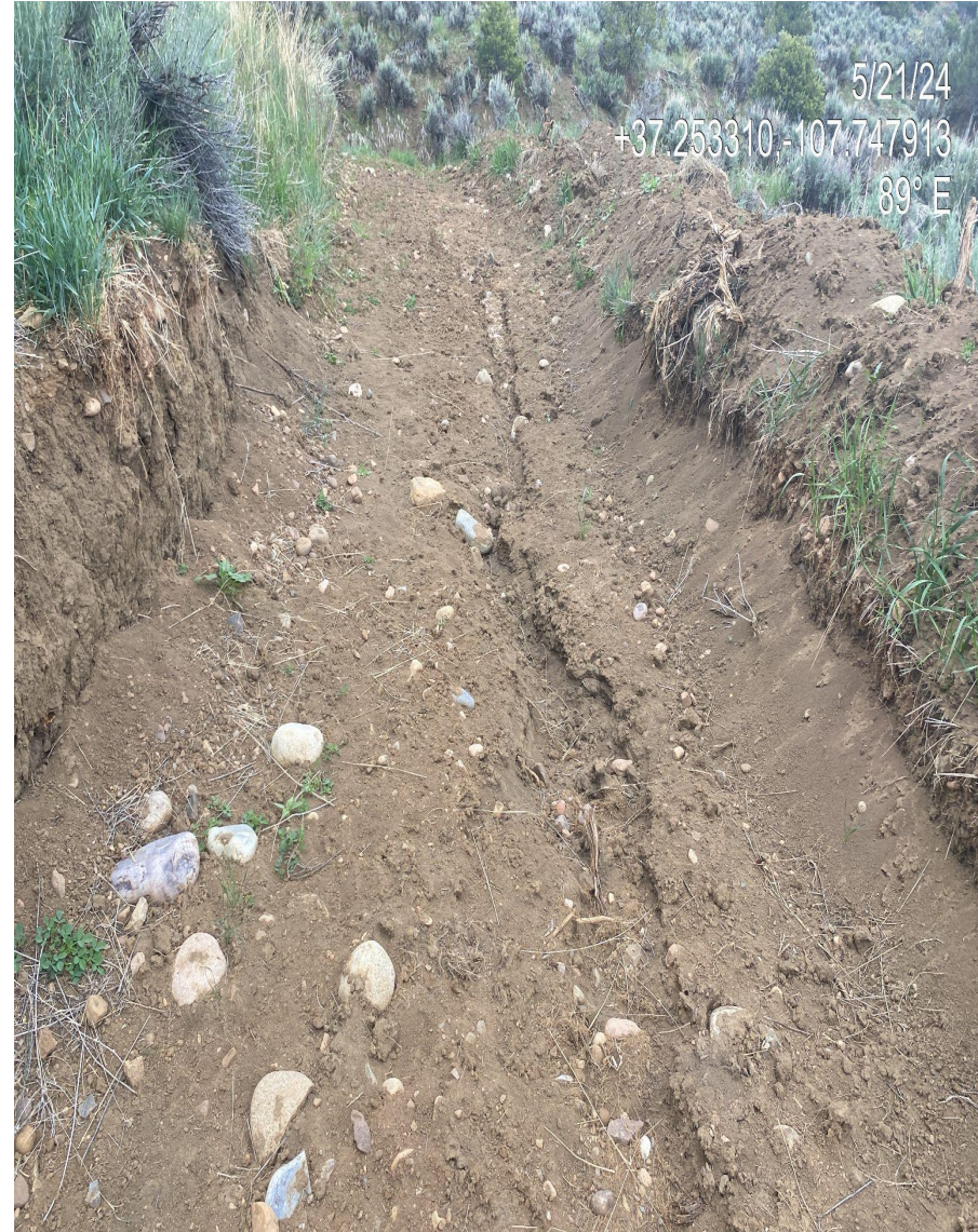
Photo 5. New storm water divergent channel has not been installed per good engineering practices. Rill erosion and evidence of sediment transport persists, additional stabilization is needed in this area.
