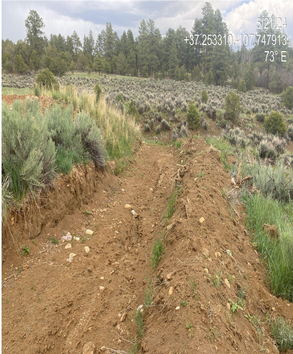
Photo 5. New storm water divergent channel has not been installed per good engineering practices. Rill erosion and evidence of sediment transport persists, additional stabilization is needed in this area.
