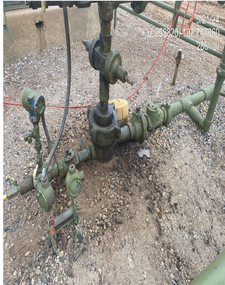
Photo 6. Impacted surface material observed at the pump jack muffer and well head.
