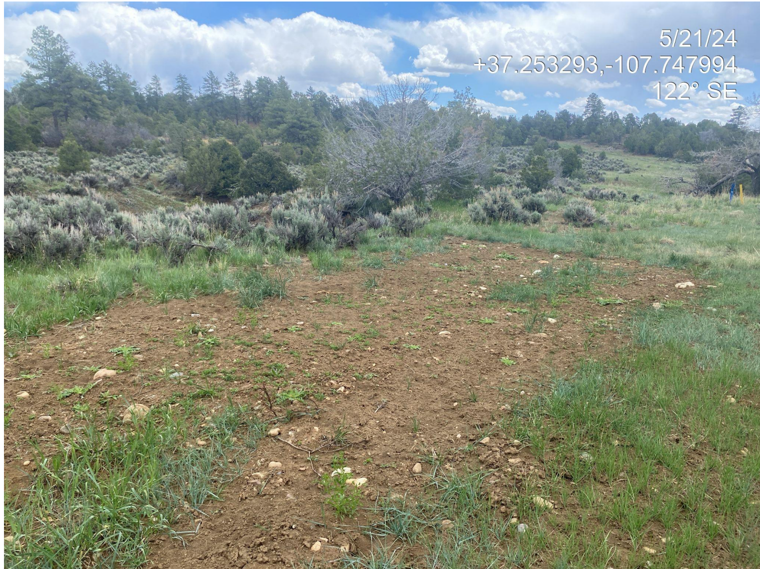
Photo 4. View of gully erosion identified in previous inspection doc that has been collapsed, regraded and reseeded. Germination of western wheatgrass observed.
