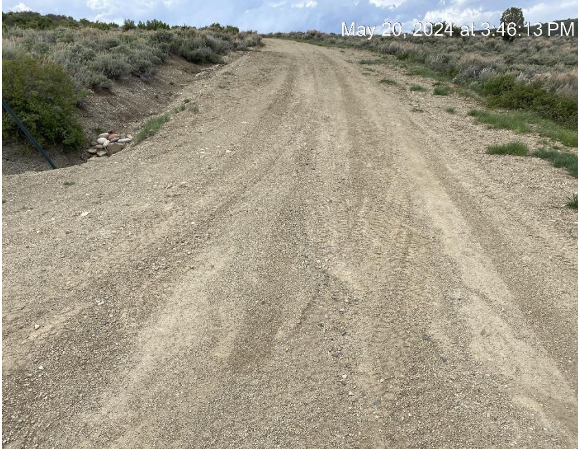
Lack of Stormwater BMP maintenance.
