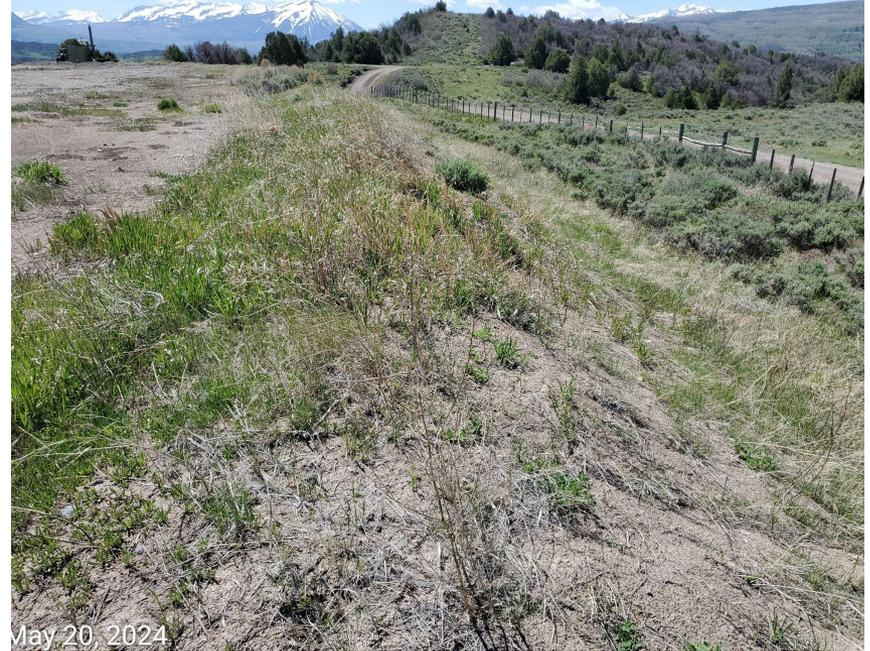
**Photo 2:** Photos examples showing fill slopes on the Location; interim reclamation to reduce the Location to areas only needed for production has not been performed in accordance with 1003 Rules.
