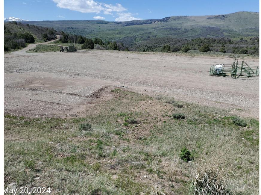
**Photo 1:** Photos 1-2 taken from the east end of the Location. Photos provide an overview of the Location from south, southwest, northwest to north. Photos also show interim reclamation to reduce the Location to areas only needed for production has not been performed in accordance with 1003 Rules.
