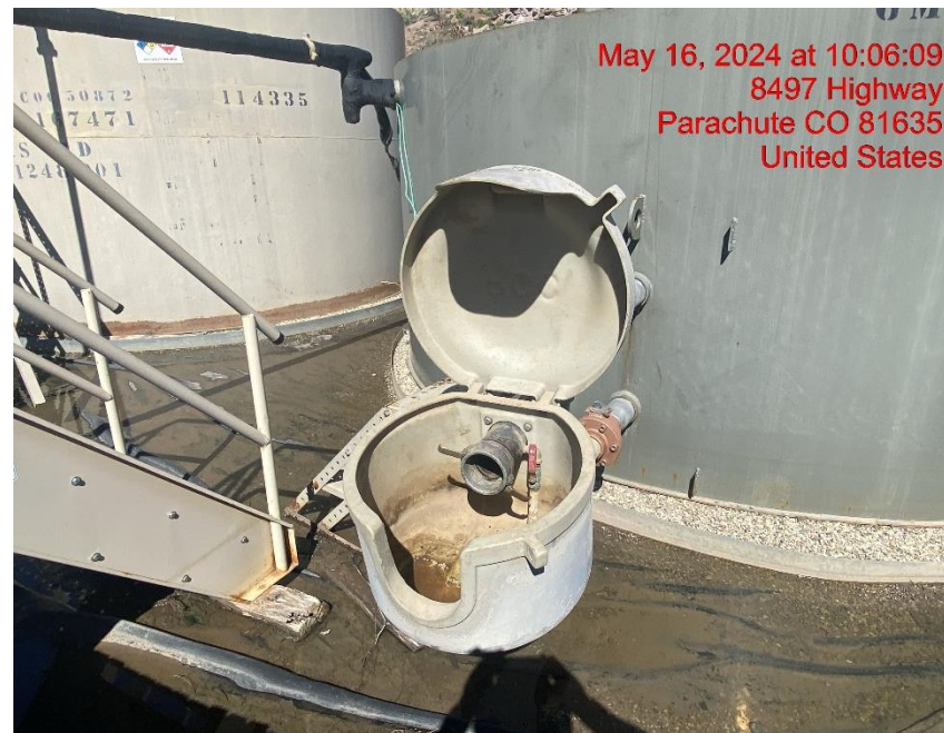
Open-Ended Load Line – Photo #01242
