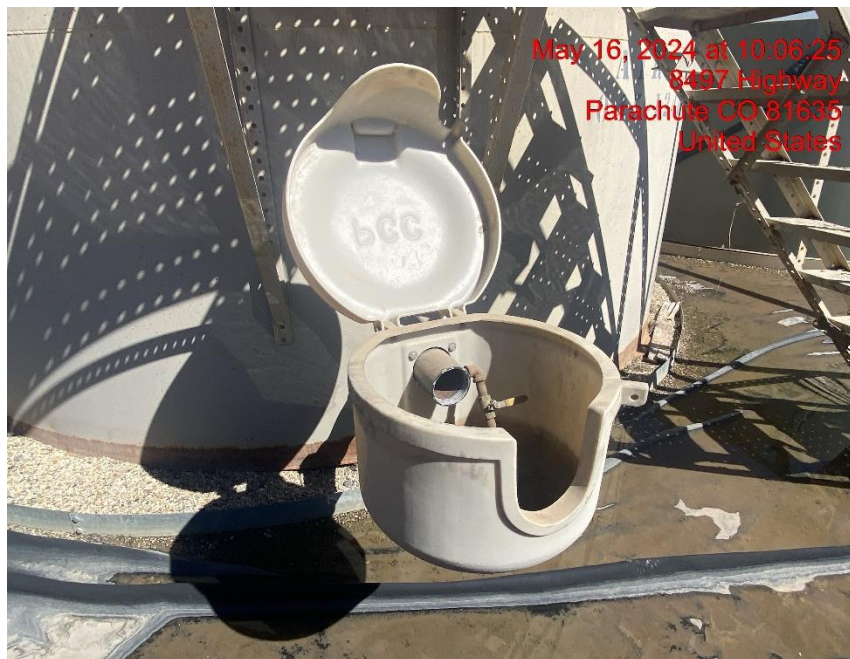
Open-Ended Load Line – Photo #01243
