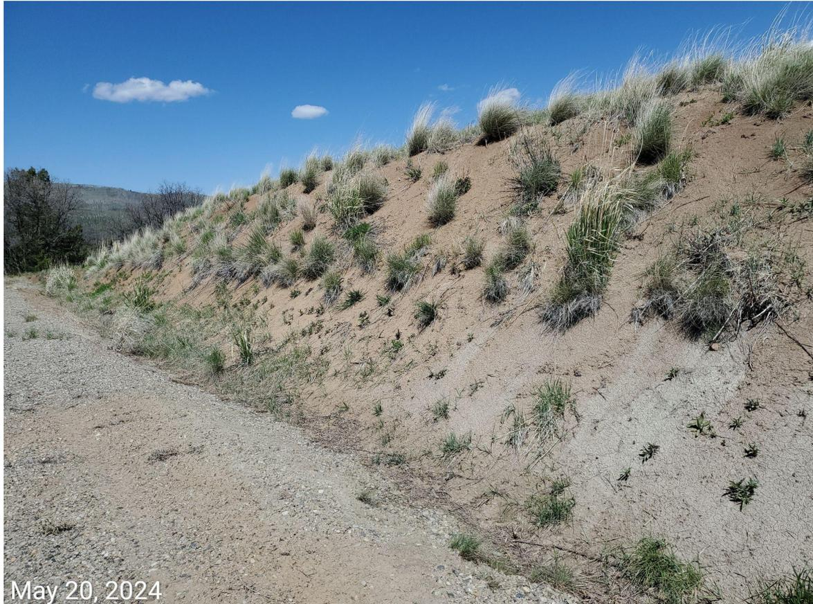
**Photo 3:** Photo taken from the Topsoil stockpile on the northwest end of the Location. BMPs to stabilize soils are missing or insufficient; soils are bare and at risk to wind and water erosion.
