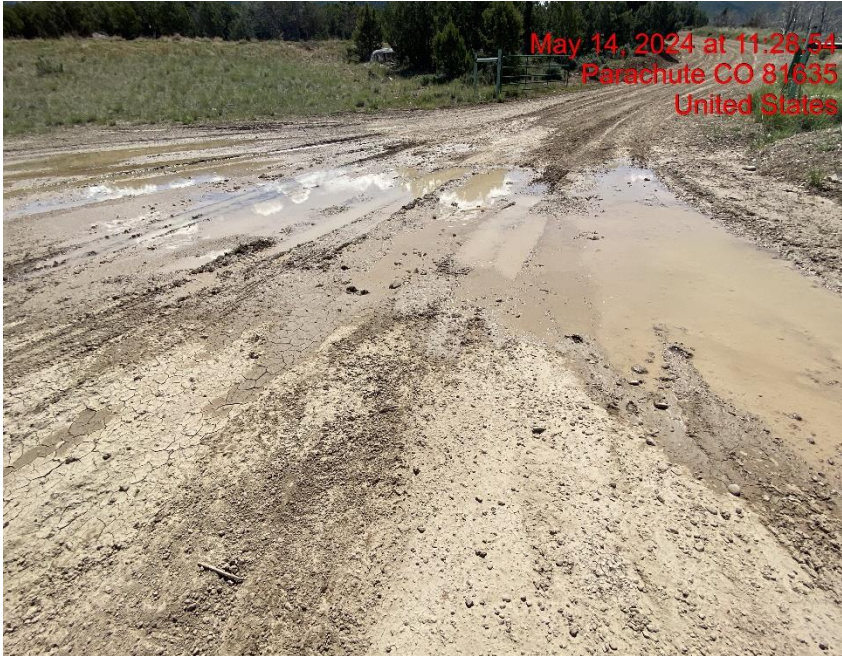
Lack of Stabilization/Insufficient Vehicle Tracking BMPs at Location Entrance/Exit – Photo #01225
