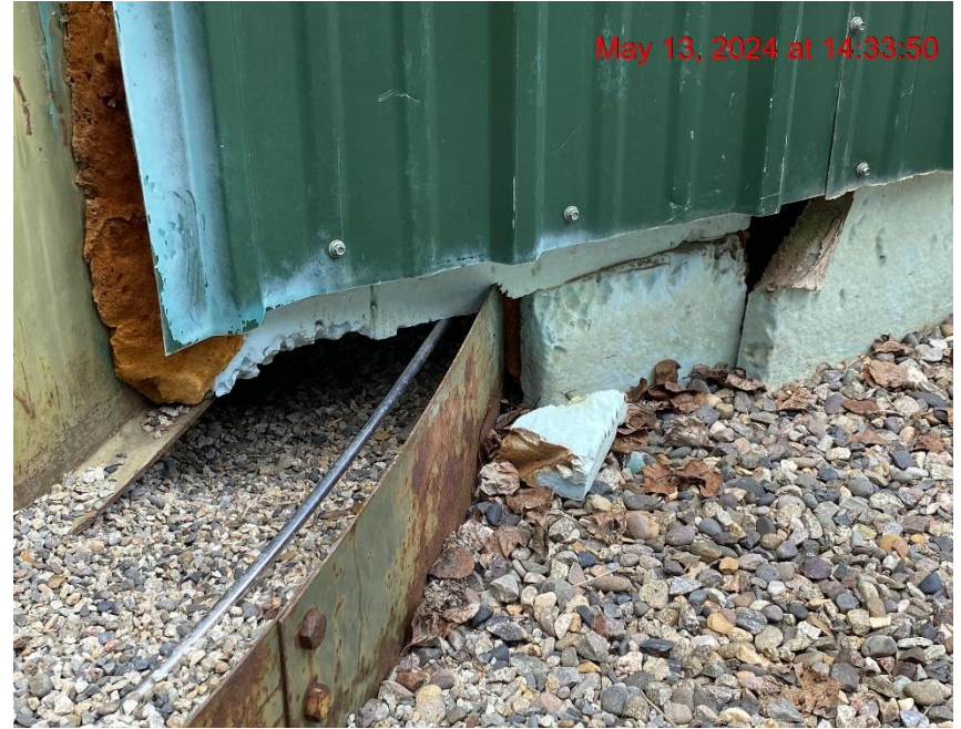
Wildlife Entry Hazard at Load Line Housing – Photo #01214
