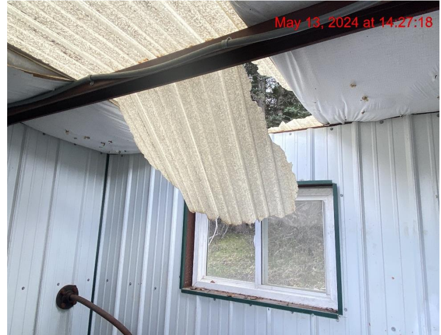
Pump House Roof Damage – Photo #01208
