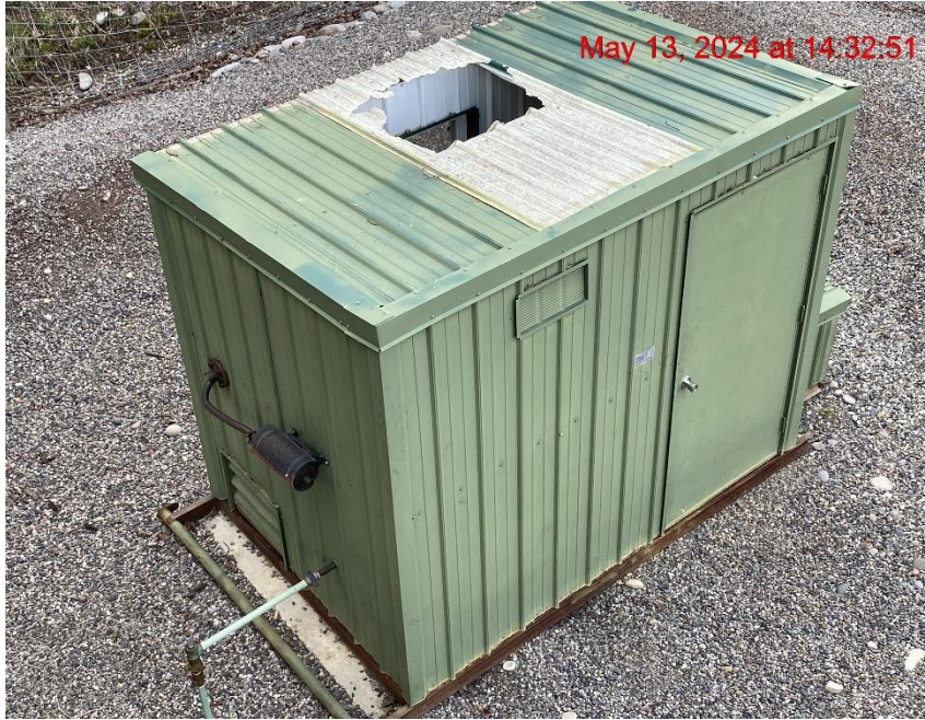
Pump House Roof Damage – Photo #01213
