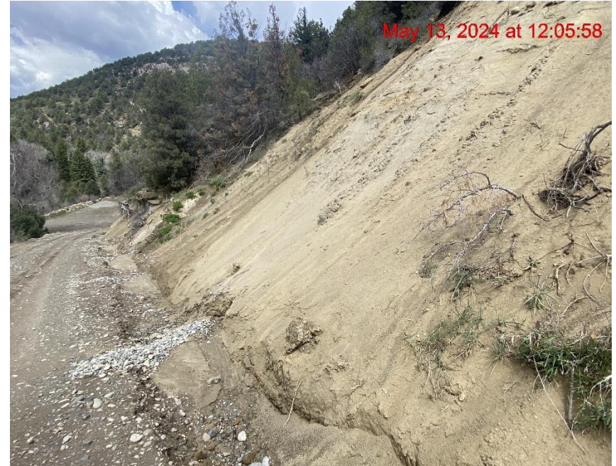
Insufficient Erosion Controls/BMP Needs Maintenance on Lease Road – Photo #01131
