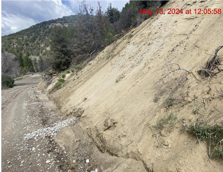
Insufficient Erosion Control/BMP Needs Maintenance on Lease Road – Photo #01131
