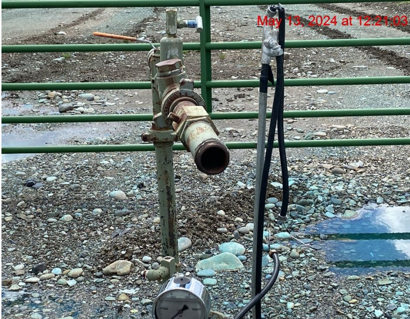
Open-Ended Line on Wellhead – Photo #01140
