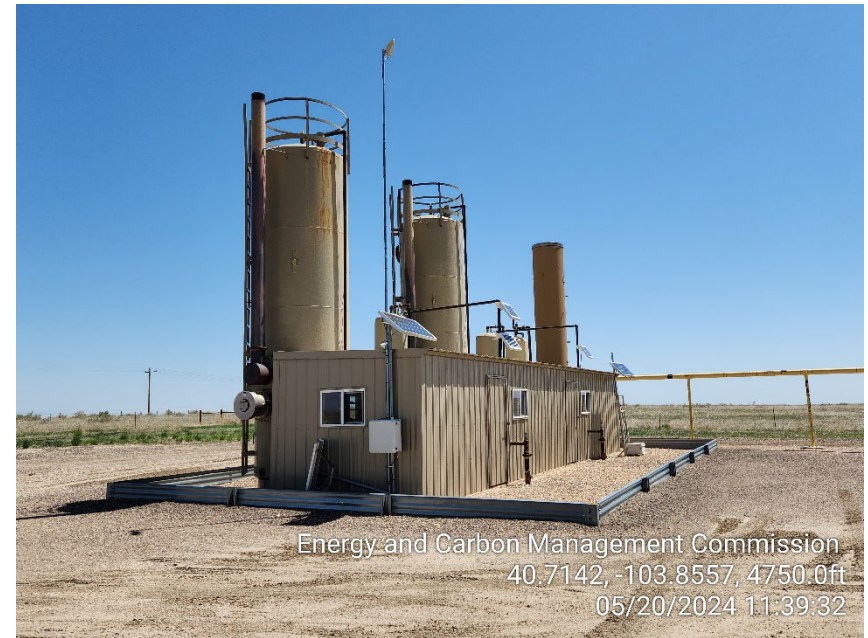
Photo 2 – Heater Treaters and ECD
