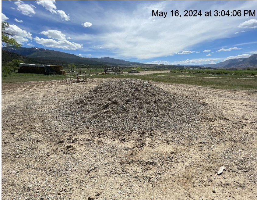
Photo # 7502 Stockpiled soils with no BMP's
