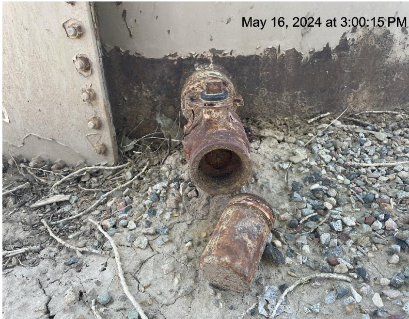
Photo # 7496 Open ended load line
