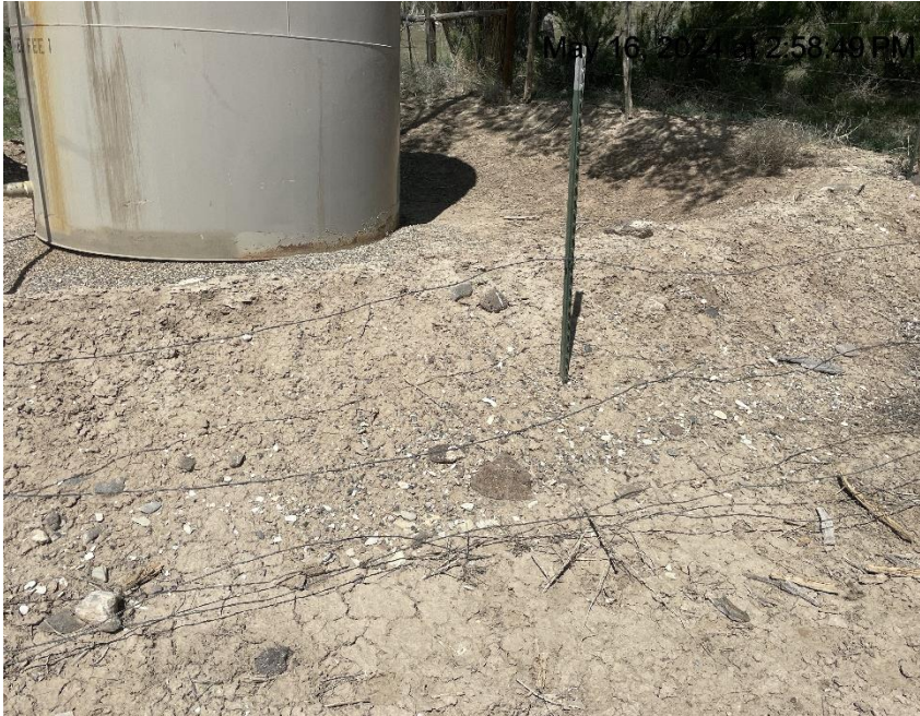
Photo # 7500 Wire fencing around tank battery needs maintenance
