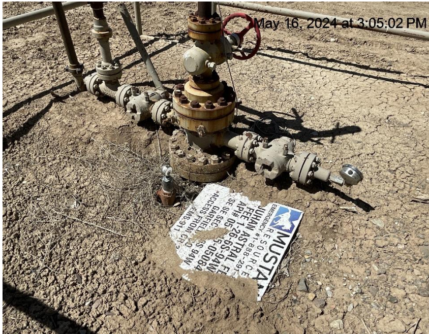
Photo # 7498 Wellhead sign not properly posted
