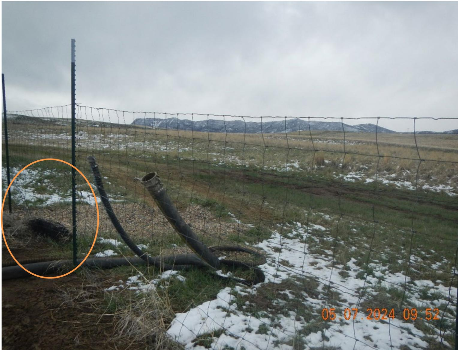
Facility #116587 REM 28244 Photo #16. hoses going through fence on west side. Appears that fluid was being removed from this side of the pit. Note: gaps in fence (in orange circle)
