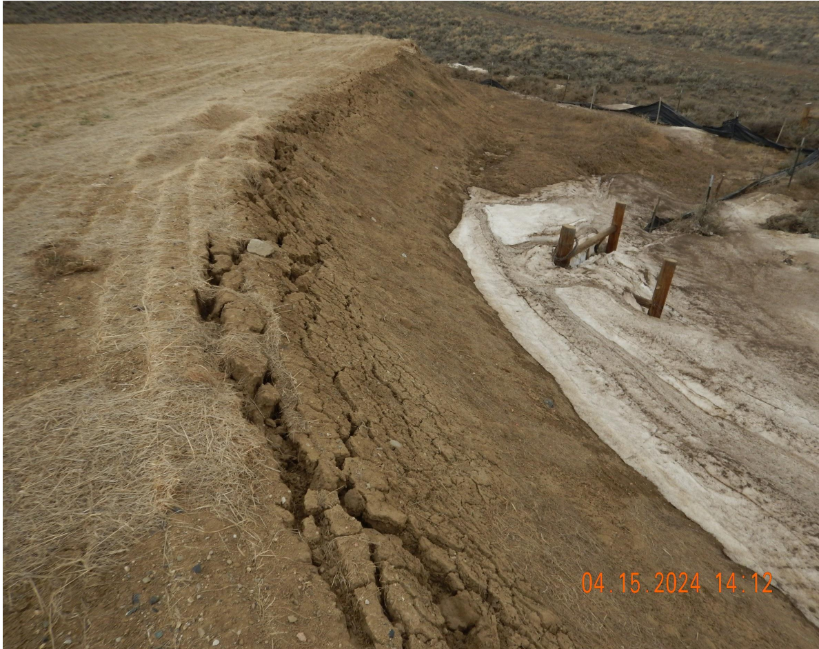
Photo 3. Photo taken from the eastern location, facing North. Photo illustrates the topsoil stockpile has not been properly stabilized and is eroding due to vertical slopes. The perimeter BMP does not appear to be an appropriate BMP given the snow accumulation in the winter months, which will continue to cause failures.
