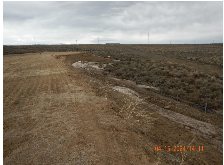
Photo 2. Photo taken from the eastern location, facing North. Photo illustrates the topsoil stockpile which has not been properly stabilized and the perimeter BMP has not been maintained.
