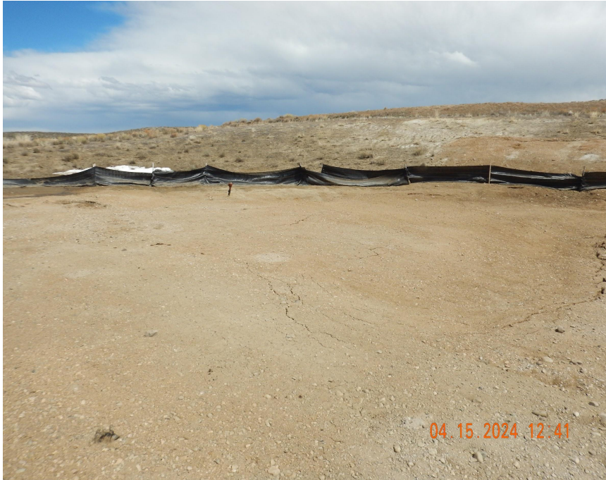
Photo 4. Photo taken from the location, facing East. Photo illustrates the silt fence BMP is in disrepair and has not been properly installed.
