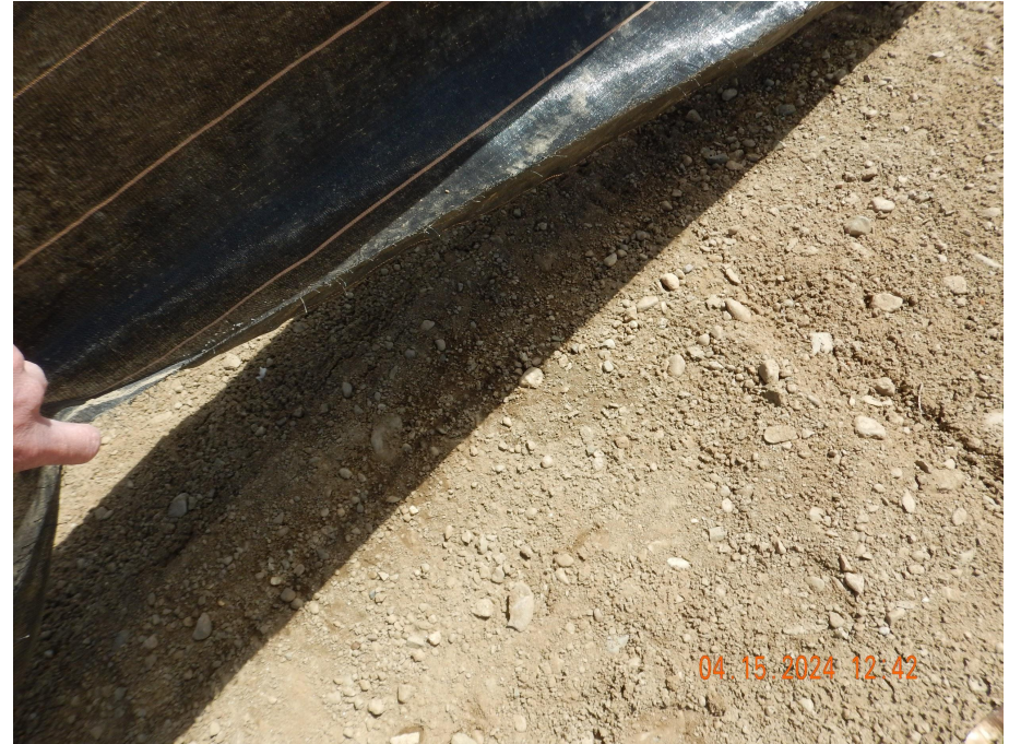
Photo 5. Close up photo taken of the improperly installed silt fence BMP.
