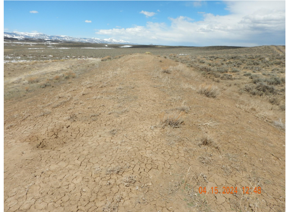
Photo 9. Photo taken from the topsoil stockpile, facing North. Photo illustrates the topsoil stockpile has not been properly stabilized for long-term stabilization.
