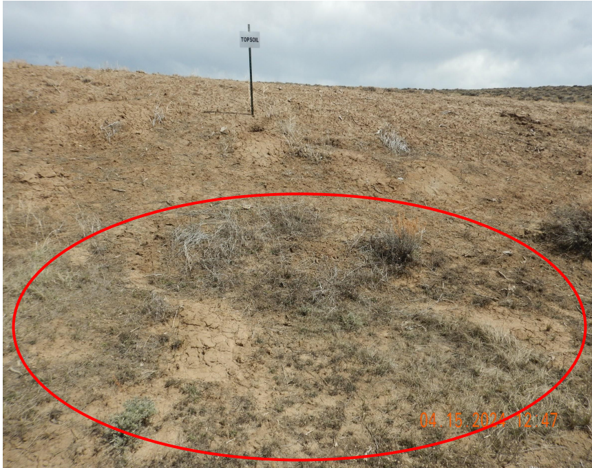
Photo 8. Photo taken from the eastern interim reclamation area, facing East. Photo illustrates the topsoil stockpile which is not properly stabilized with evidence of erosion without a perimeter BMP.
