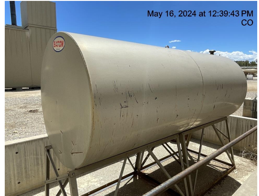
Photo # 7431 Tank lacks required labeling
