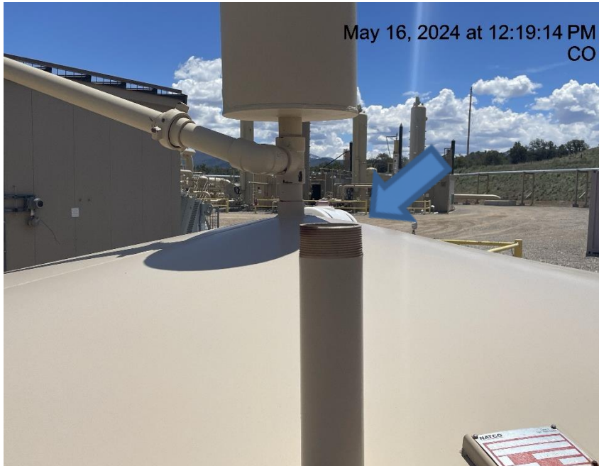
Photo # 7416 Open ended piping on VRU tank/wildlife hazard
