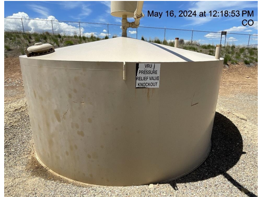
Photo # 7415 VRU tank lacks required labeling
