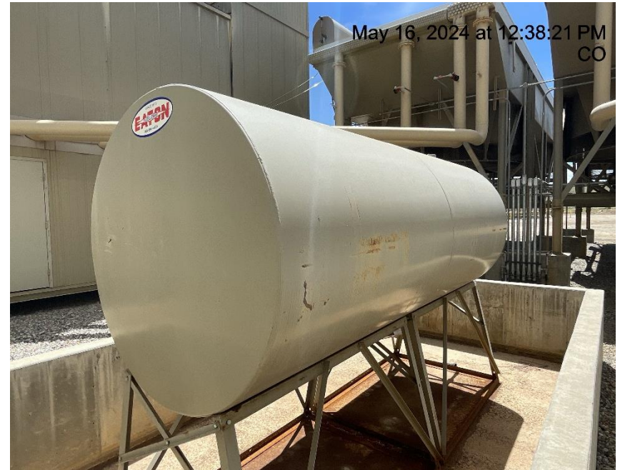
Photo # 7429 Tank lacks required labeling
