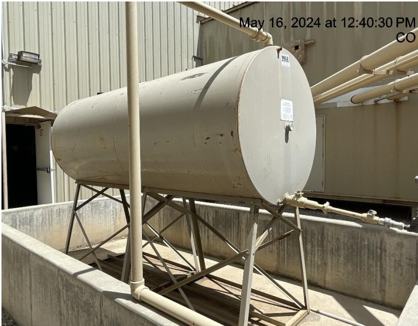
Photo # 7432 Tank lacks required labeling
