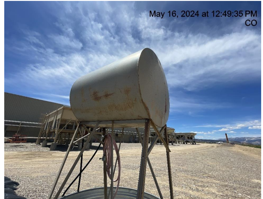
Photo # 7423 Diesel tank lacks required labeling
