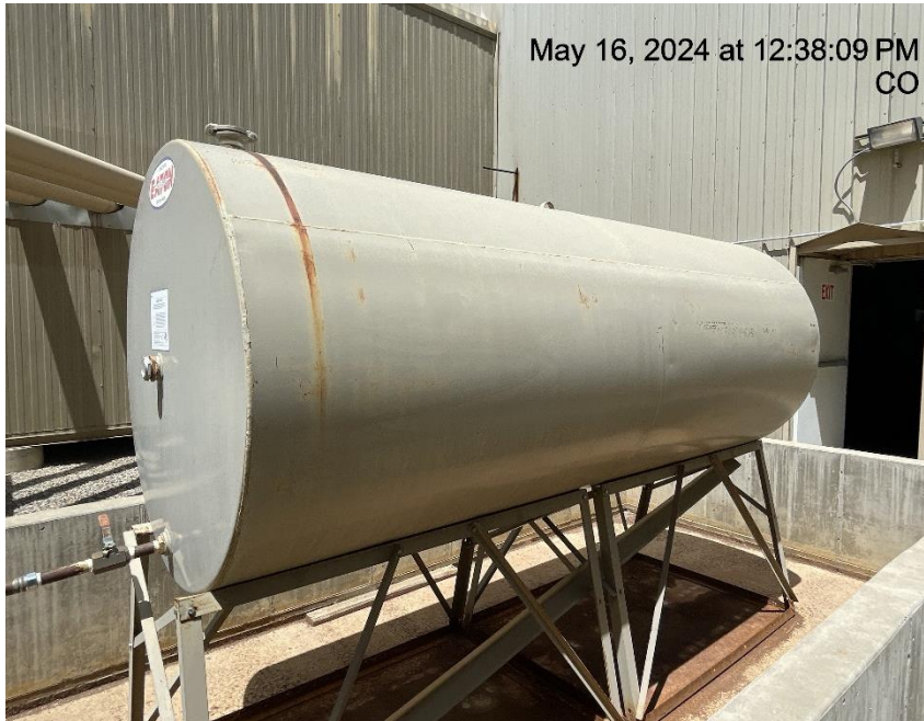
Photo # 7428 Tank lacks required labeling
