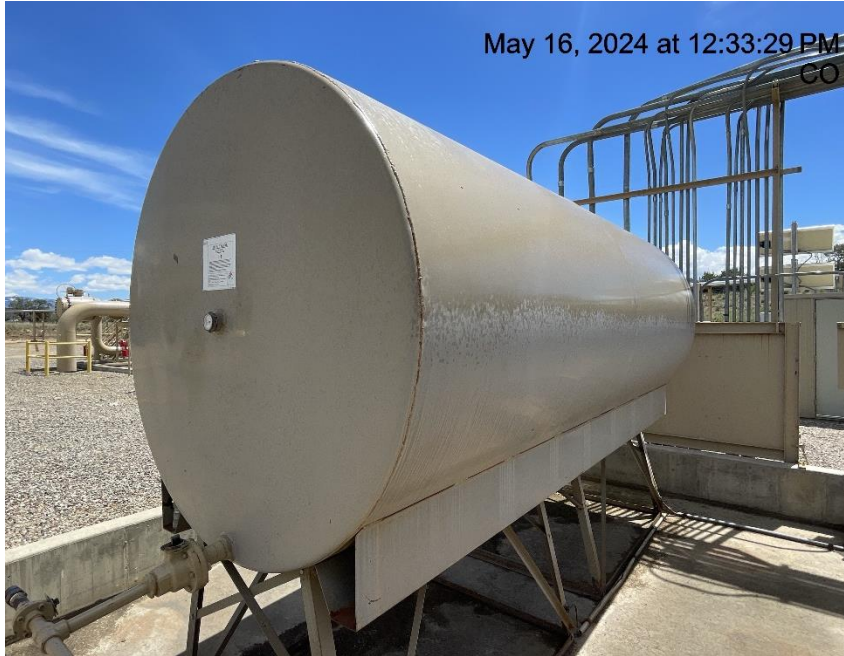
Photo # 7424 Tank lacks required labeling
