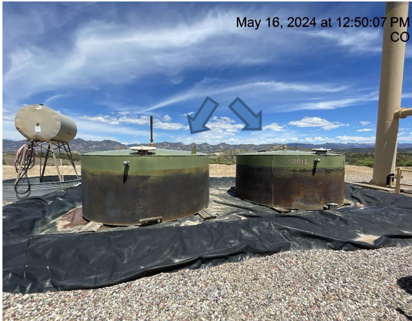
Photo # 7418 Tanks lack required labeling
