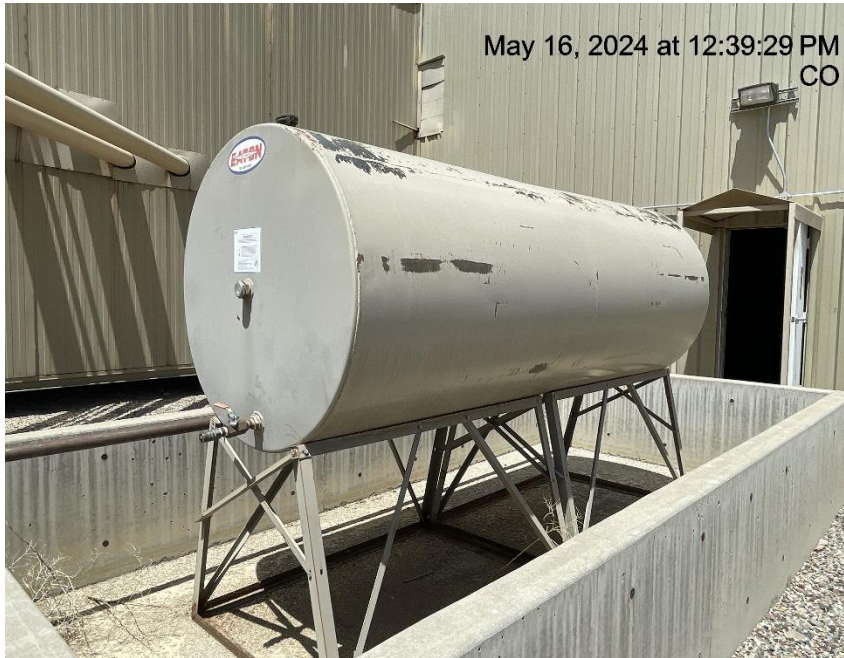
Photo # 7430 Tank lacks required labeling
