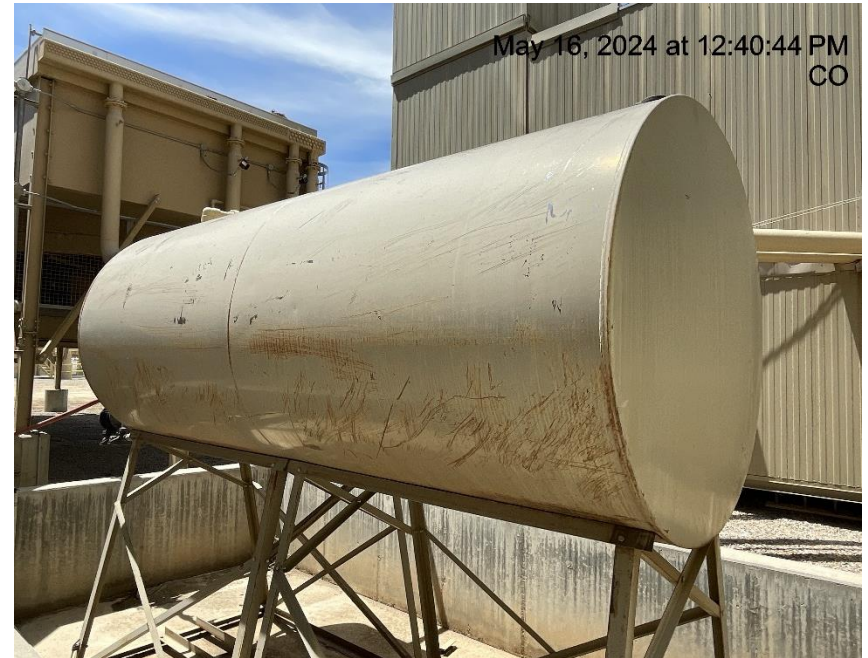
Photo # 7433 Tank lacks required labeling
