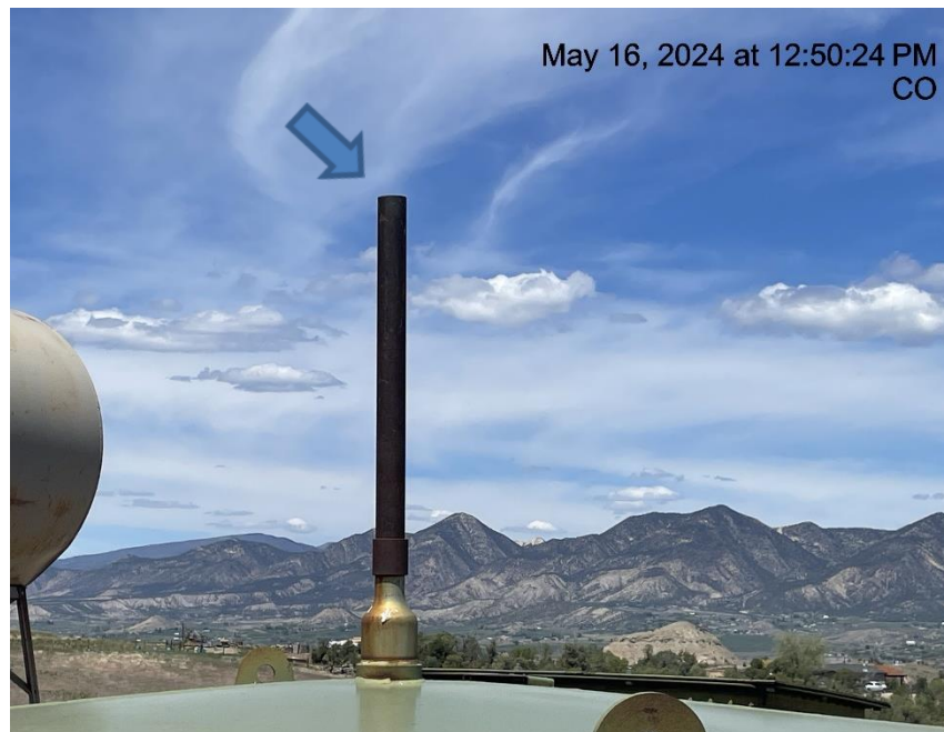
Photo # 7420 Open ended piping on tank/wildlife hazard
