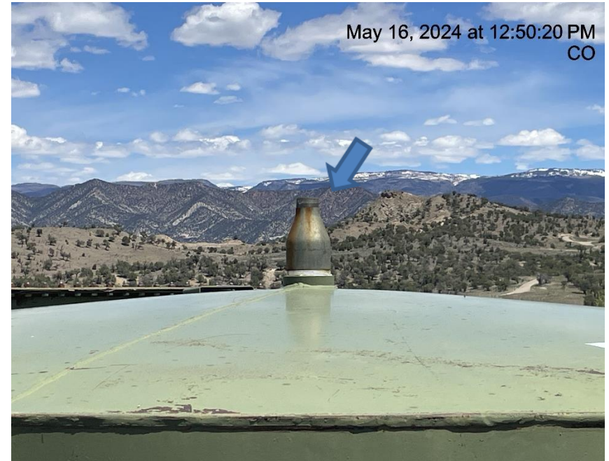
Photo # 7419 Open ended piping on tank/wildlife hazard
