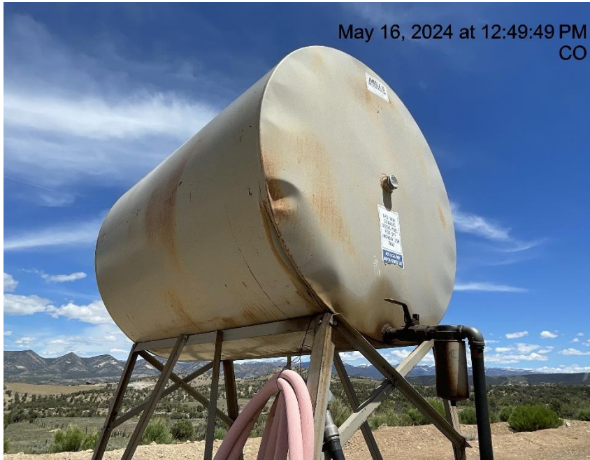
Photo # 7422 Diesel tank lacks required labeling
