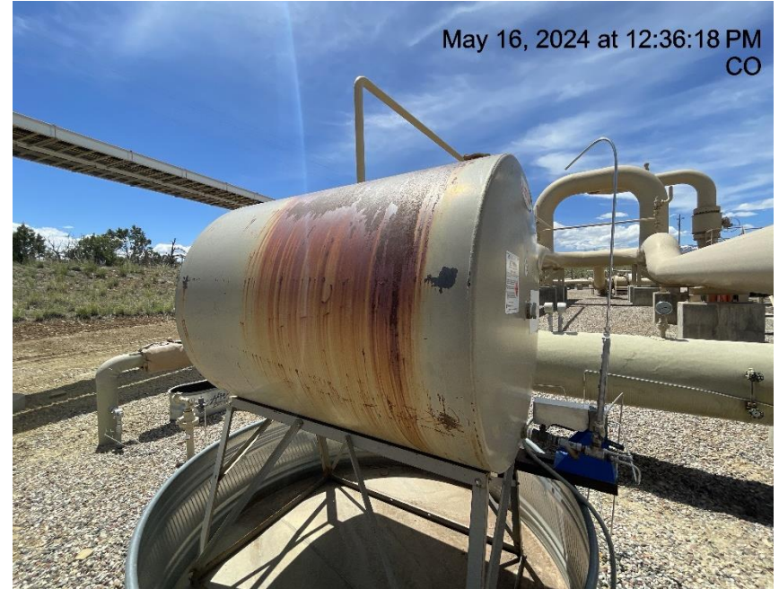
Photo # 7427 Methanol tank lacks required labeling
