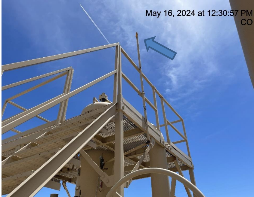
Photo # 7412 PRV vent line cap blown off/vent line does not comply with CECMC pressure safety device rules
