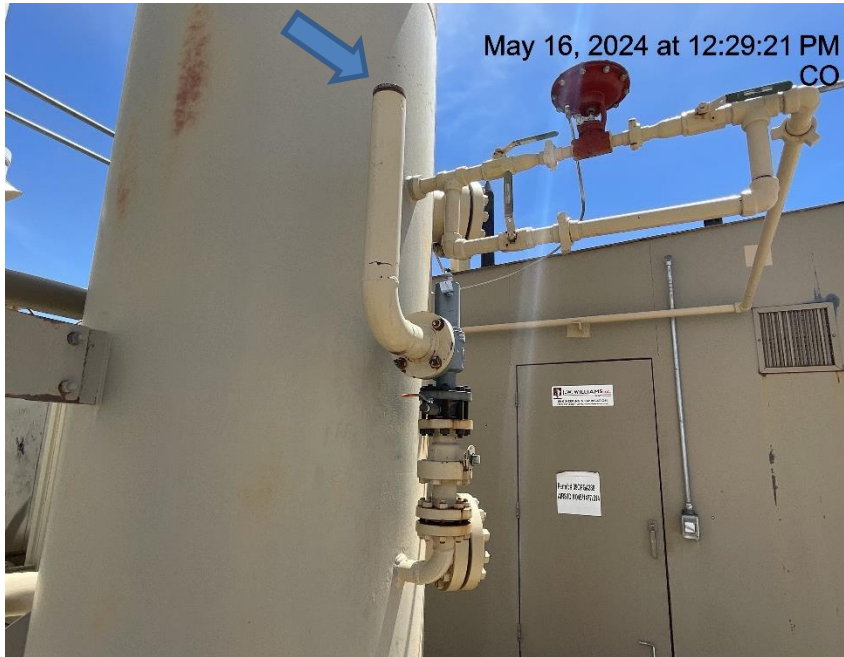
Photo # 7414 PRV vent line does not comply with CECMC pressure safety device rules
