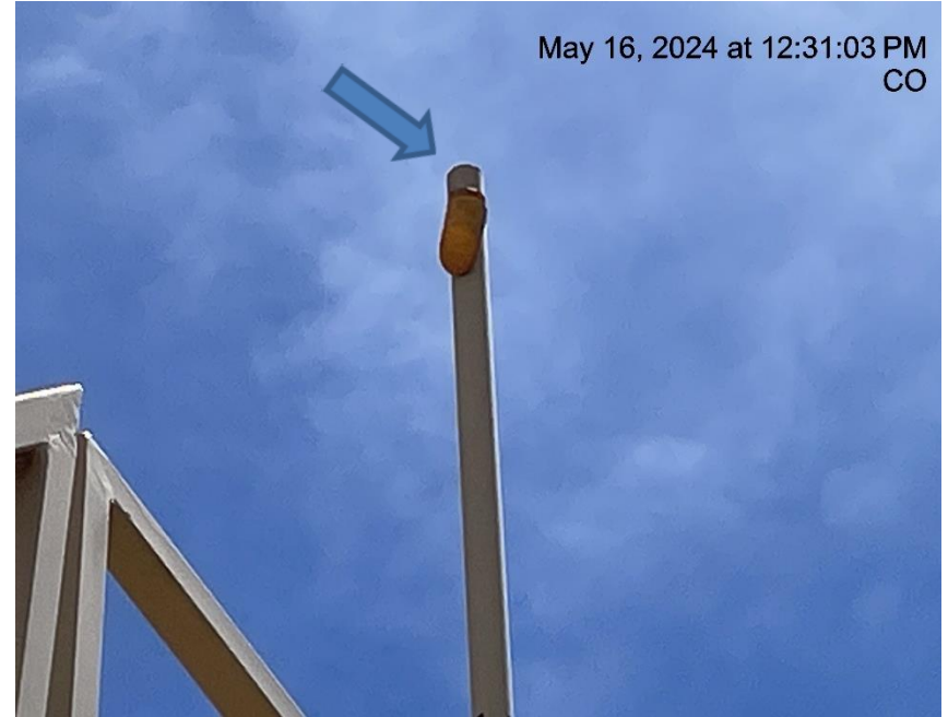
Photo # 7413 PRV vent line cap blown off/vent line does not comply with CECMC pressure safety device rules
