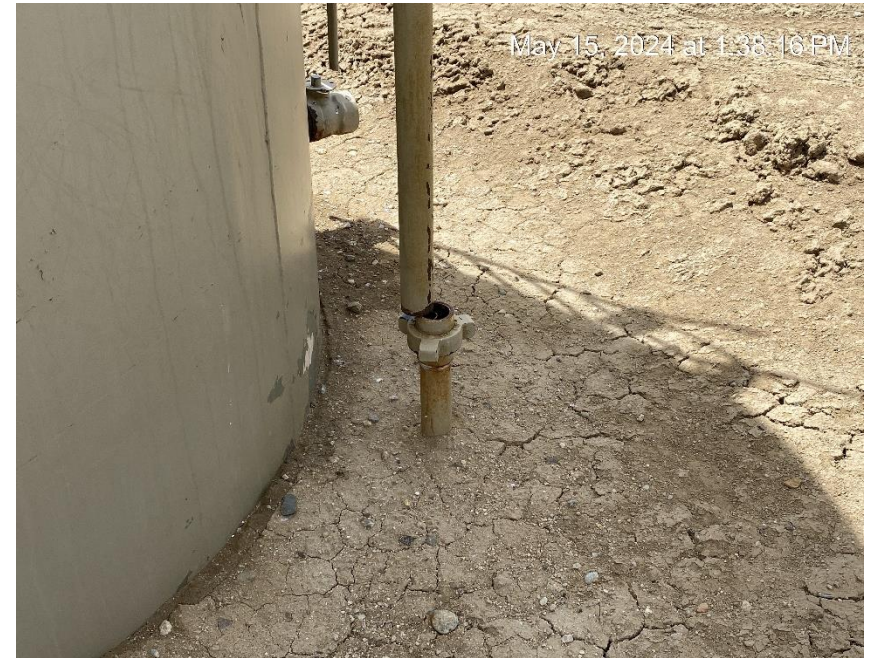
Damaged equipment. Repair or remove line.
