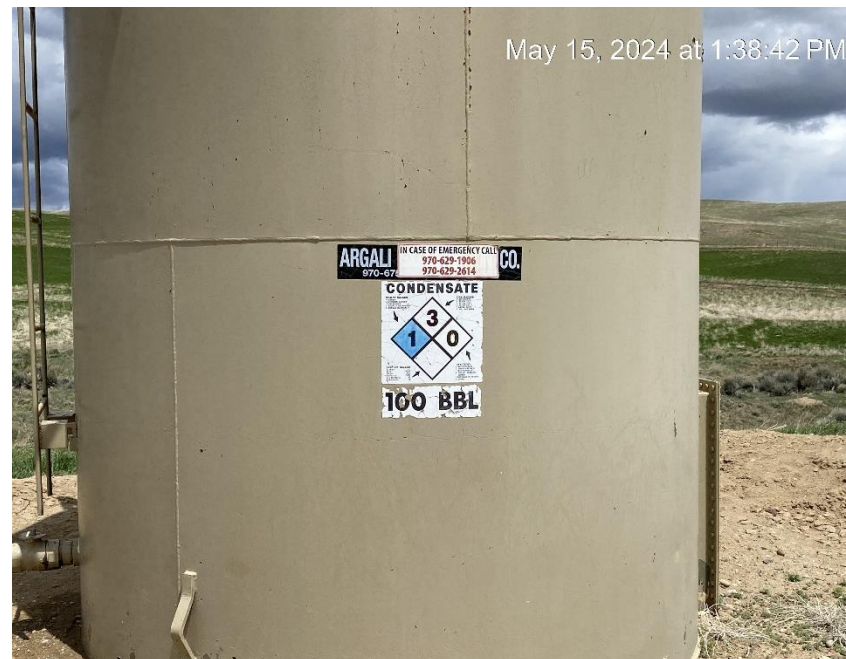
Condensate tank without proper containment next to a natural drainage area
