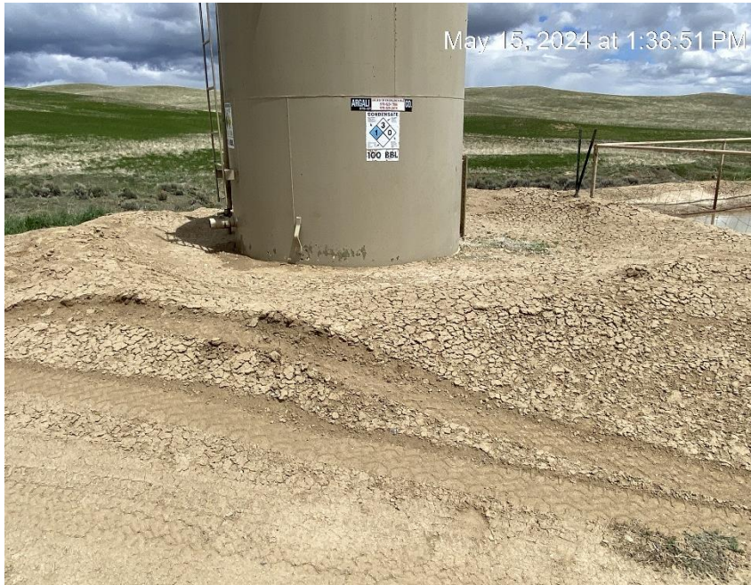
Inadequate tank berm. Natural drainage behind tank.
