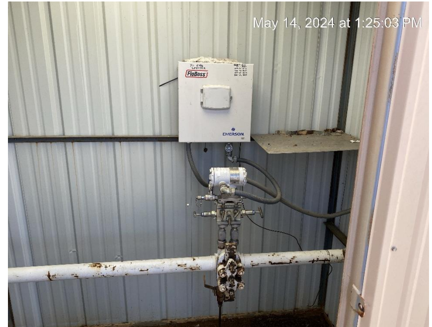
No display of gas meter calibration
