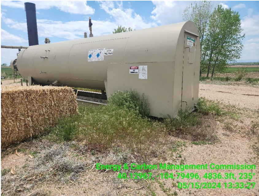
Photo 13 Vegetation around the Heater Treater need to be addressed.
