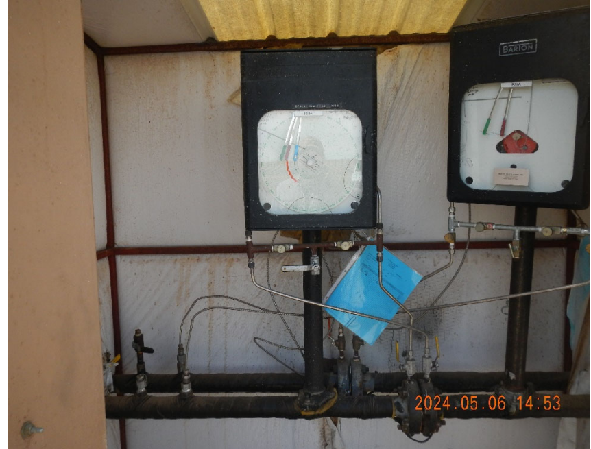
4. Gas meter inside meter shed.
