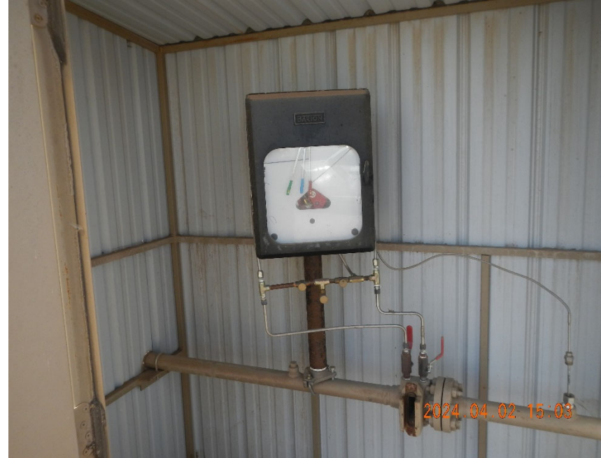
2. Gas meter inside meter shed.
