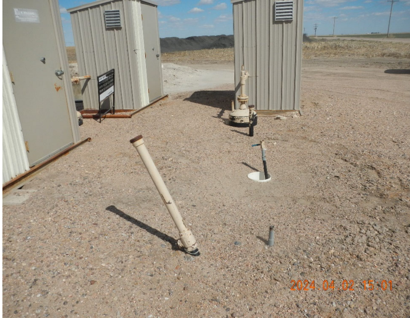
3. Flowline risers at gas meter shed.
