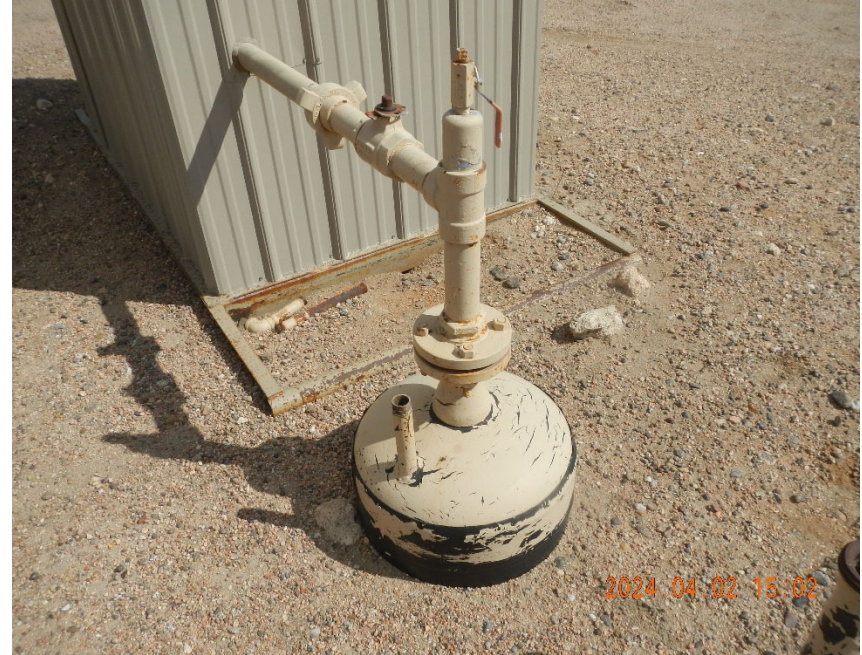
4. Partially buried gas dryer vessel at gas meter shed.
