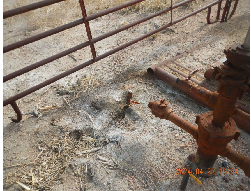
8. Damp soil and salt ring around riser with seep at valve and plug.
