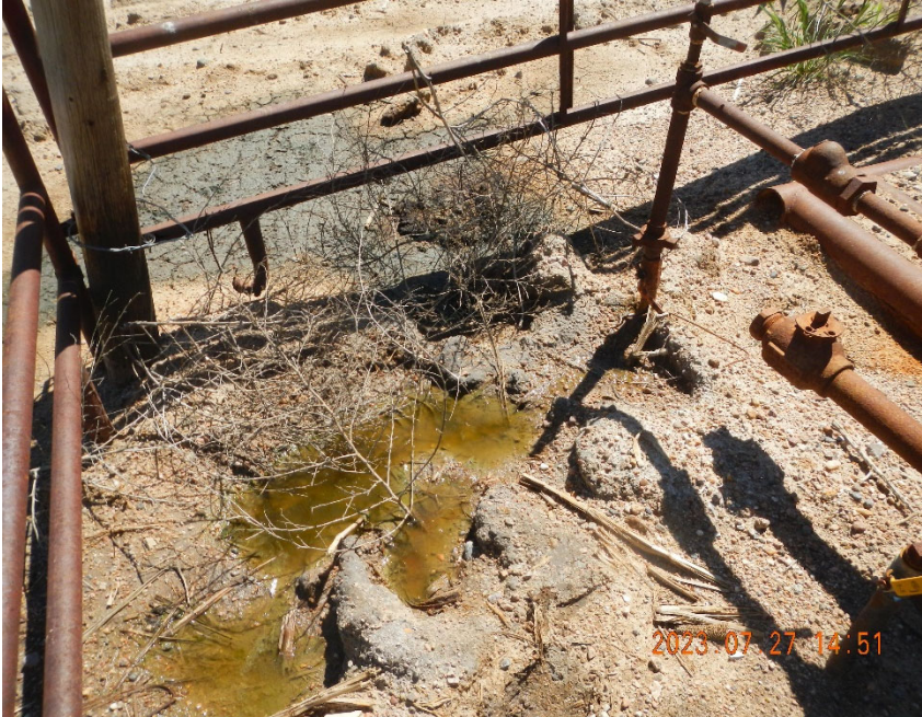
3. View of water leg leaking at valve and hammer union 7/27/2023 inspection.
