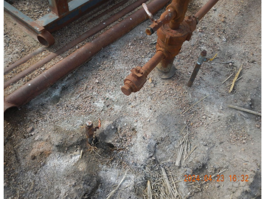
6. View of removed pipe section and fittings on water leg.
