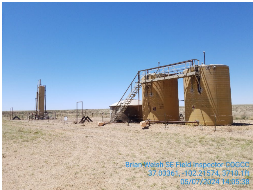
Tank battery and treater
