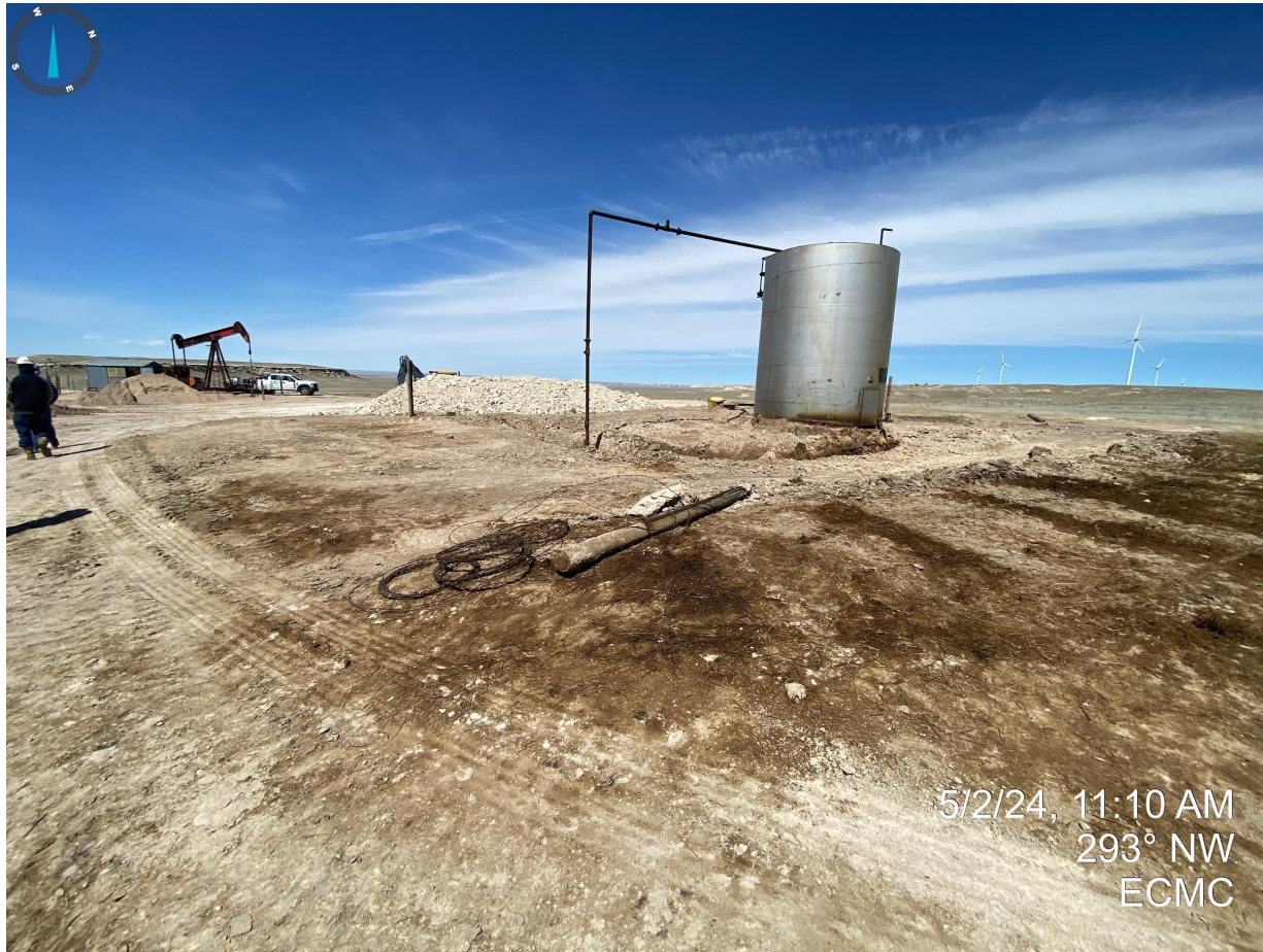
Photo 8. Hydrocarbon impacts observed east/southeast of the tank battery.
