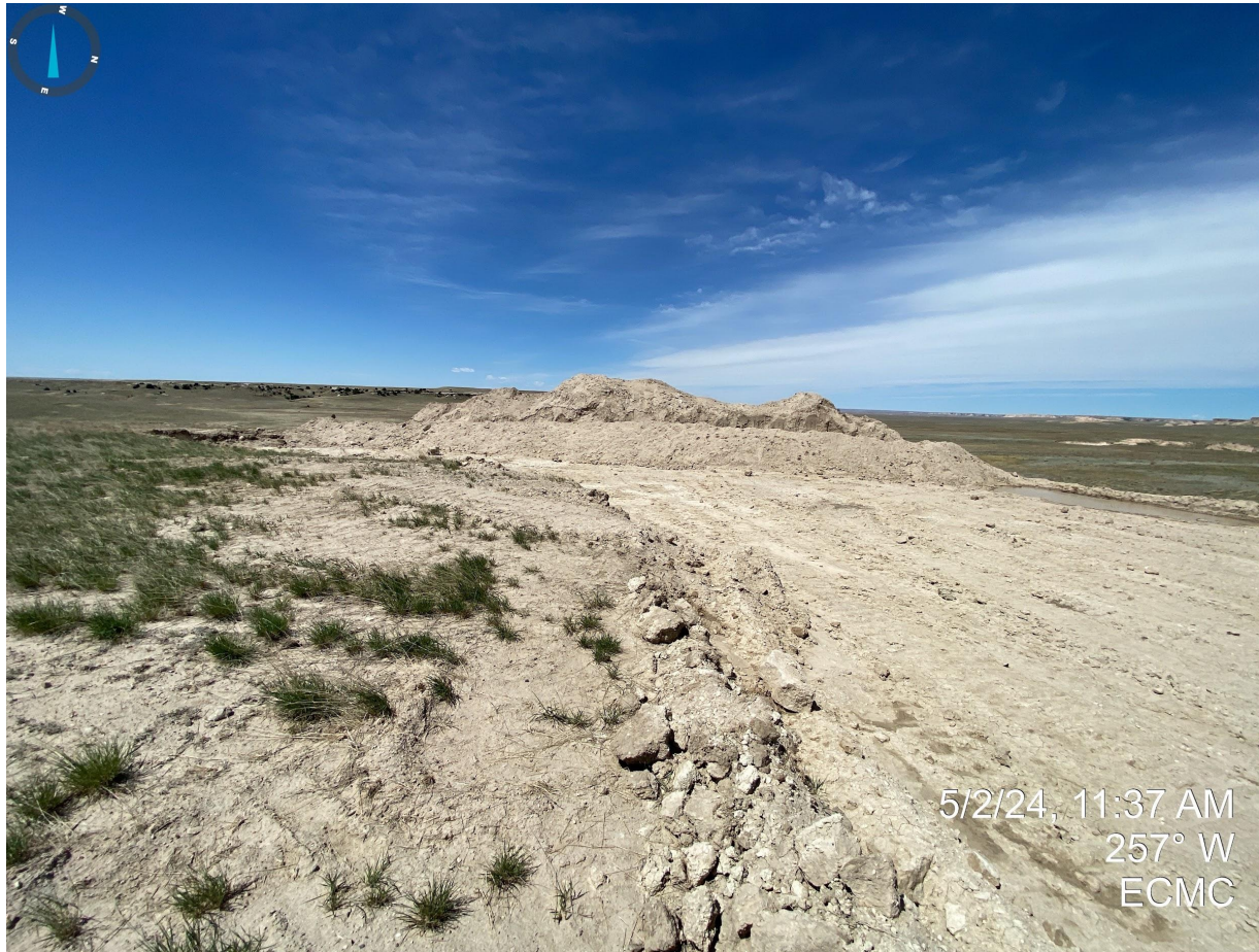
Photo 23. Overview of excavated pit and salt kill area. Soils do not appear to be properly stabilized from wind and water erosion degradation. The open excavation is not properly fenced to exclude wildlife, livestock or unauthorized personnel.
