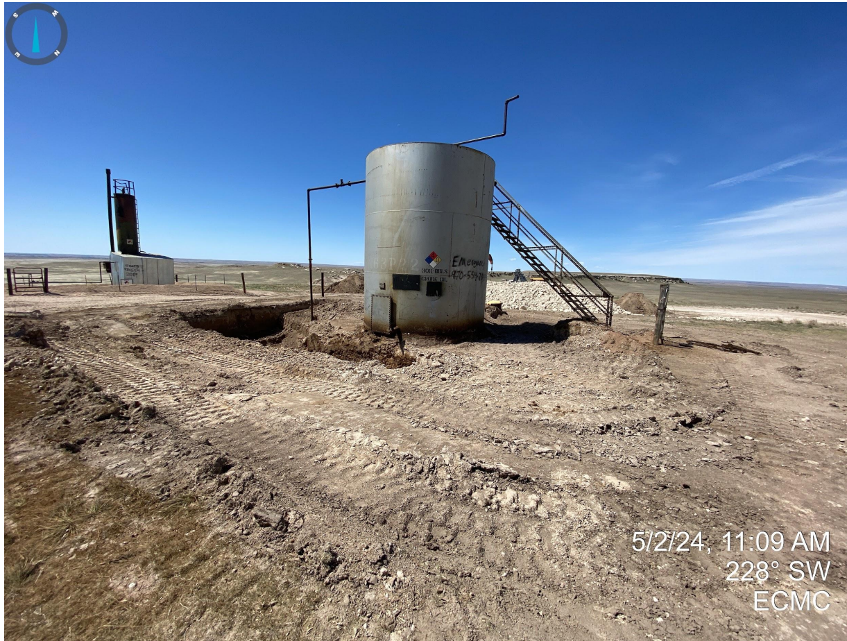
Photo 1. Free hydrocarbons previously observed within the tank battery secondary containment have been removed and the tank battery area has been excavated. Refer to Environmental FIR (doc #709100276) photo log from 04/29/2024 for additional.
