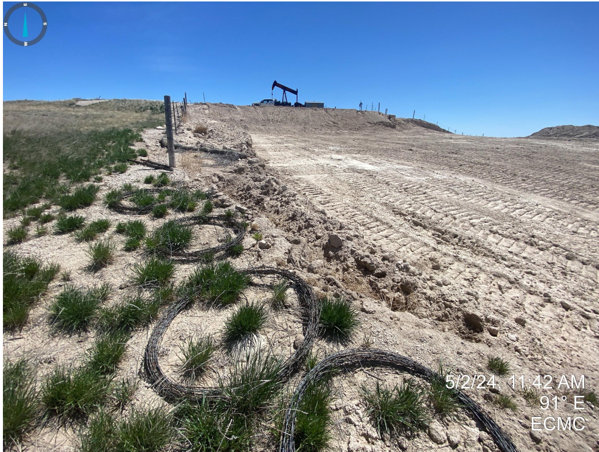
Photo 28. Unused fencing material needs to be removed from the location or returned to service as it poses a potential hazard to personnel, livestock and wildlife resources.
