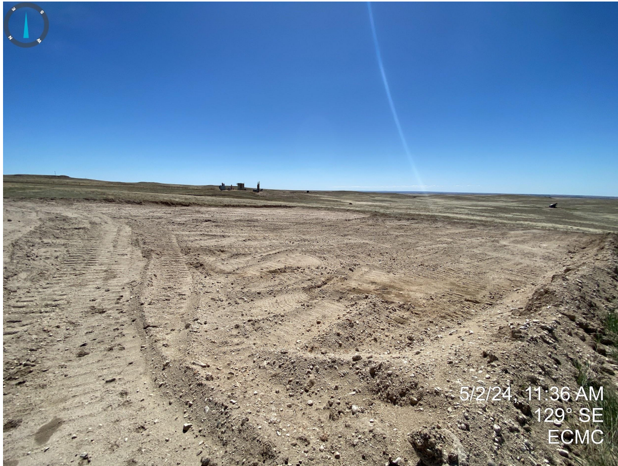
Photo 19. An area approximately 0.50 acres in size has been excavated south of the pit and stockpile. No evidence of stormwater controls measures were observed around the perimeter of the excavated salt kill impacted area.
