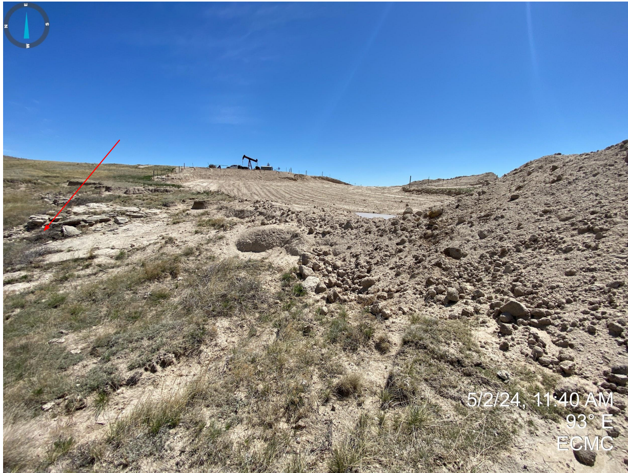
Photo 26. North side of excavation. No stormwater control measures were observed around the perimeter of the excavated area that would prevent off location stormwater discharge from entering nearby drainage (indicated by red arrow).
