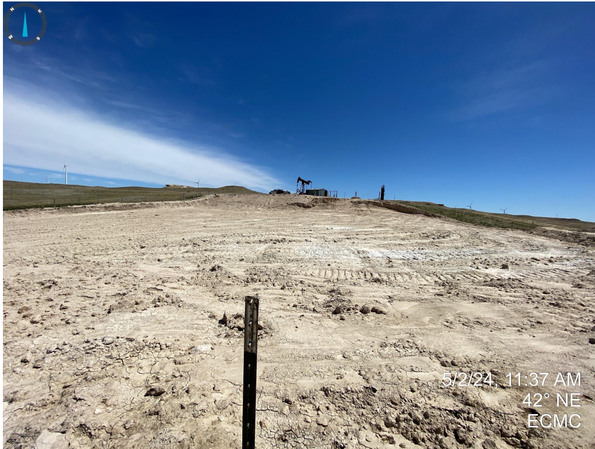
Photo 22. Overview of excavated pit and salt kill area. Soils do not appear to be properly stabilized from wind and water erosion degradation. The open excavation is not properly fenced to exclude wildlife, livestock or unauthorized personnel.
