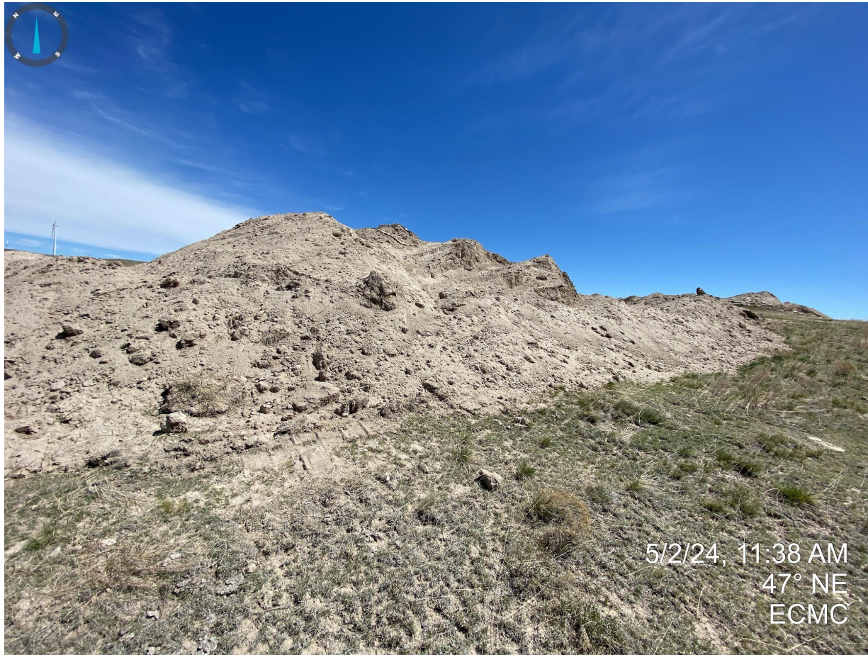
Photo 24. Western stockpiled material is not properly stabilized with evidence of unconsolidated materials.
