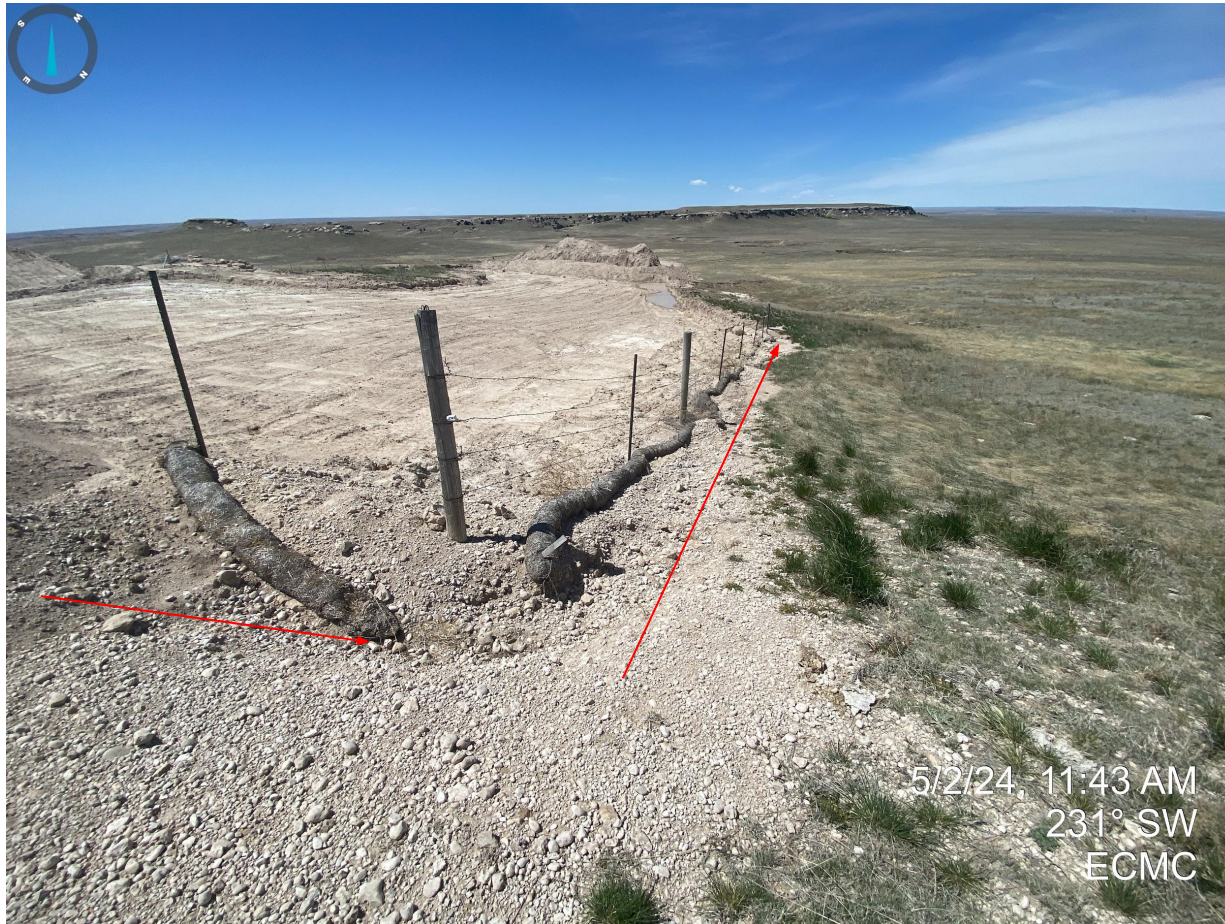
Photo 29. Taken from the north side of the pit. It does not appear that any erosion degradation has been properly stabilized or repaired, and stormwater control measure remain inadequate as the straw wattles are either degraded or not installed properly.
