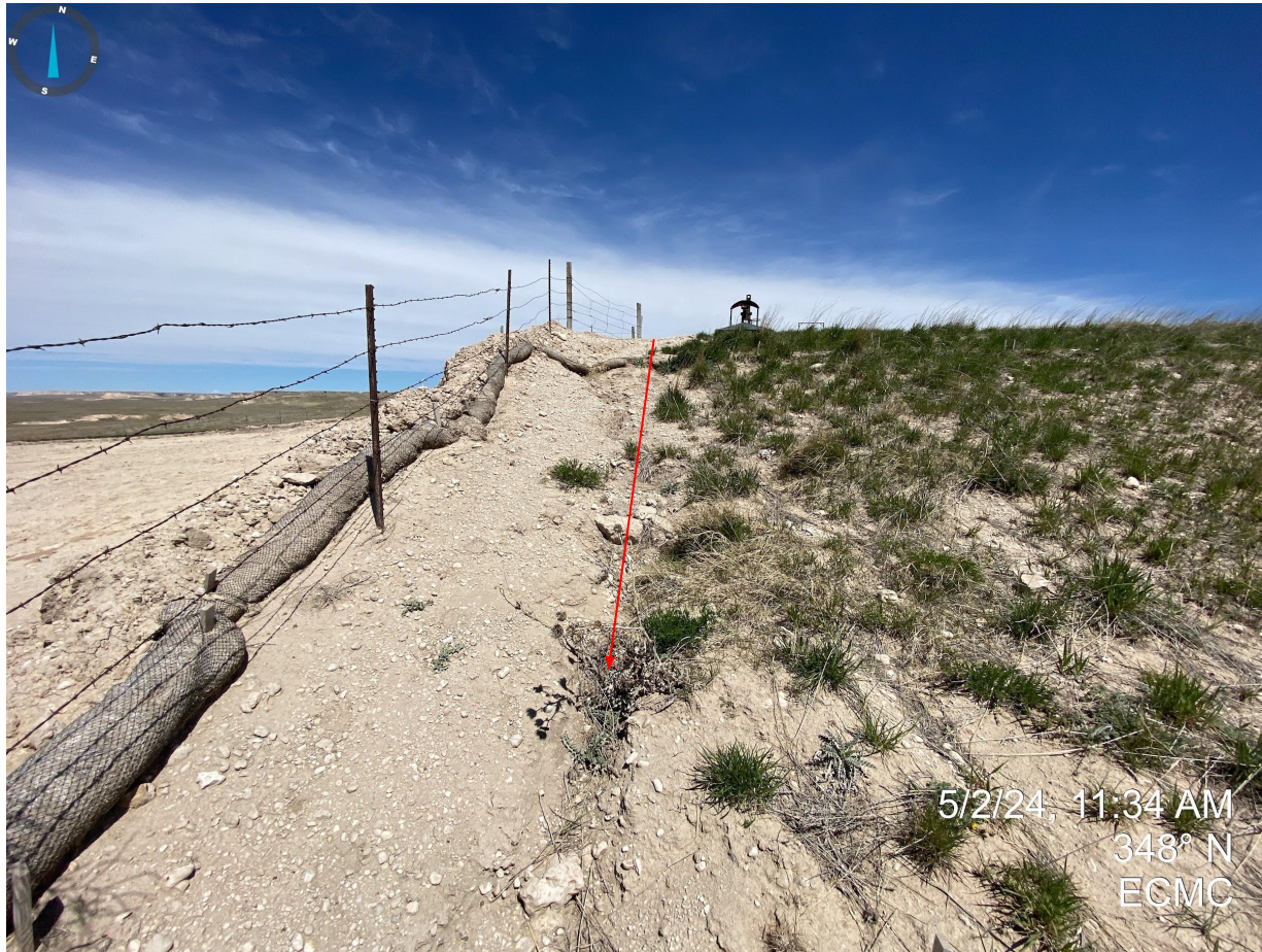
Photo 14. Erosion degradation on the east side of the pit.
