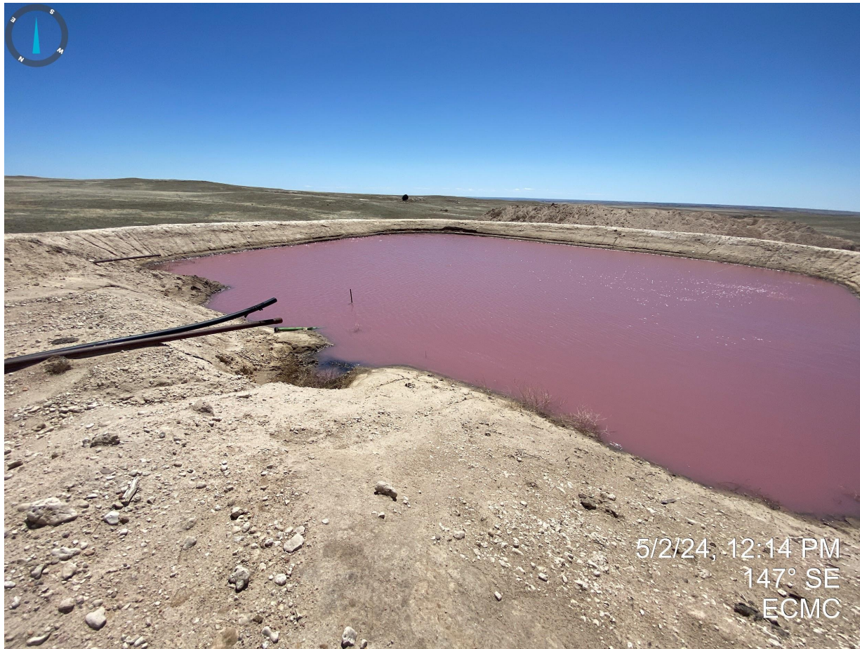
Photo 15. The produced water pit does not have adequate netting that would exclude wildlife entry.
