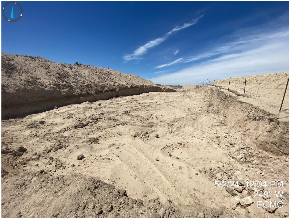
Photo 23. Photo illustrates excavated soil from the previously identified salt kill impacts. Soils within the excavation and stockpiles are not properly stabilized as they have been left unconsolidated. Unconsolidated material can become a potential source of pollution and is susceptible to wind and water erosion degradation.
