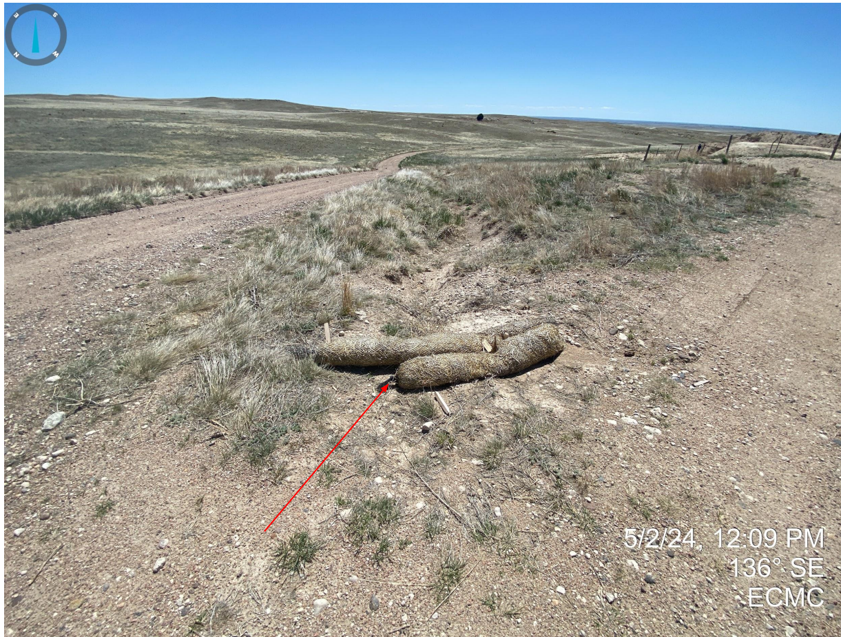
Photo 10. Stormwater control measures installed near the production areas/access road do not appear to be properly installed per good engineering practices (e.g. trenched and backfilled).
