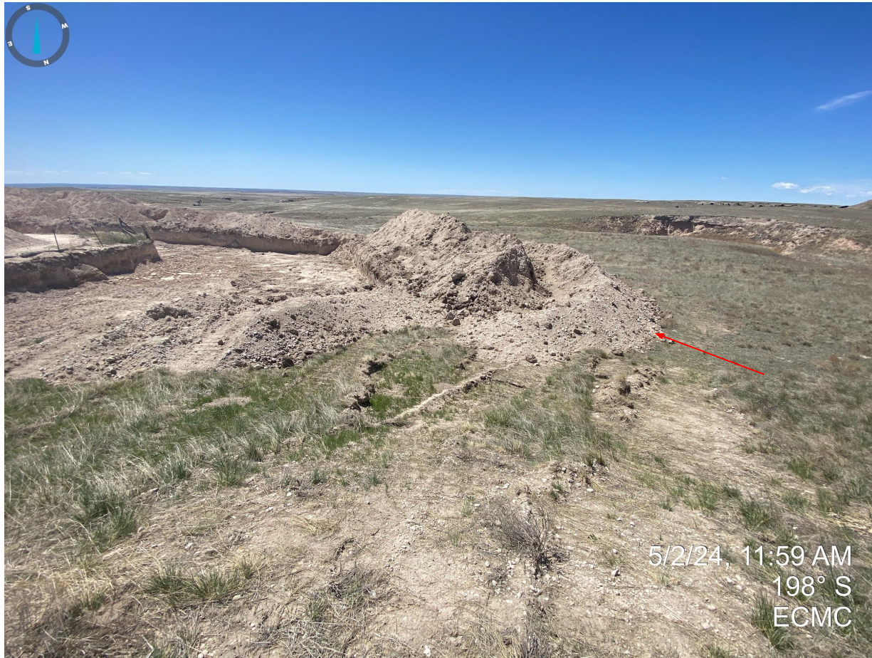
Photo 16. Taken from the north side of the stockpiled soils. No perimeter stormwater control measures/BMPs, or impermeable liners underneath the stockpile were observed during this inspection. Impacted soils appear to have been placed directly on top of undisturbed lands. Additionally, it does not appear that topsoil has been salvaged Per Rule 1002.b prior to stockpiling the soil on undisturbed portions of land.
