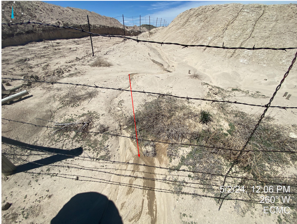
Photo 24. Taken from the southeastern portion of the pit. Photo illustrates erosion degradation on the pit walls and inadequate stormwater control measures around the base, or perimeter, of the pit.
