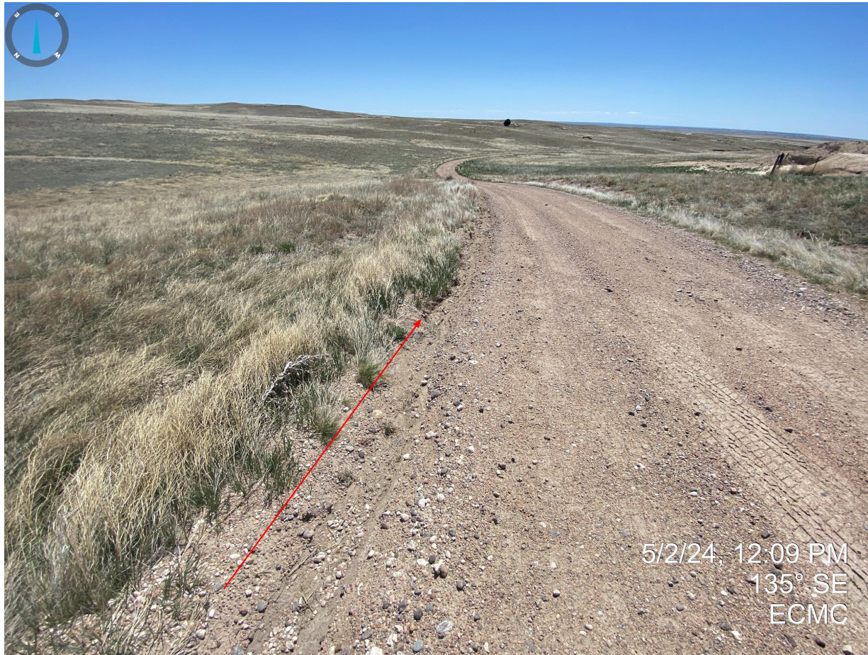
Photo 4. Taken from the access road east of the pit. Evidence of erosion degradation, previously documented, does not appear to have been repaired/stabilized with no evidence of control measures/BMPs observed that would prevent further erosion of the access road.
