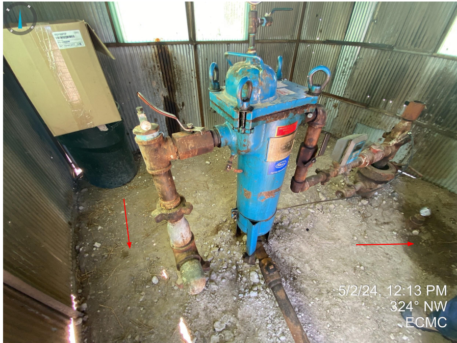
Photo 13 & 14. Stained soil observed within the injection well shed.
