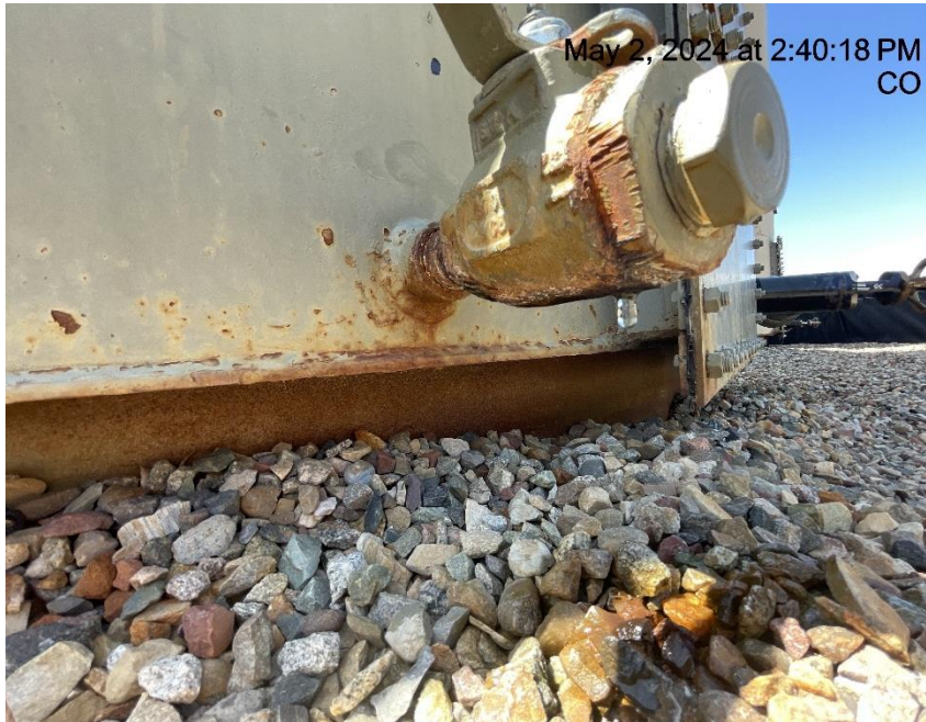
Photo # 5657 Valve on production tank leaking fluid
