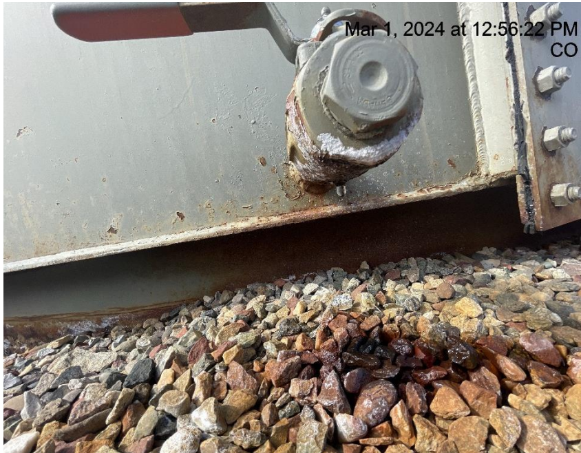
Photo # 8080 From inspection 708903187 conducted on 03/01/2024 Valve on production tank leaking fluid
