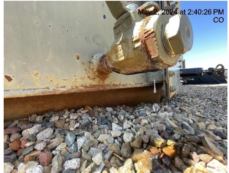
Photo # 5658 Valve on production tank leaking fluid
