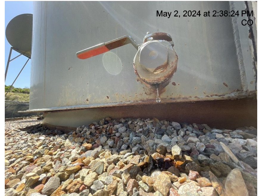
Photo # 5656 Valve on production tank leaking fluid
