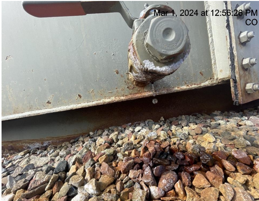
Photo # 8081 From inspection 708903187 conducted on 03/01/2024 Valve on production tank leaking fluid
