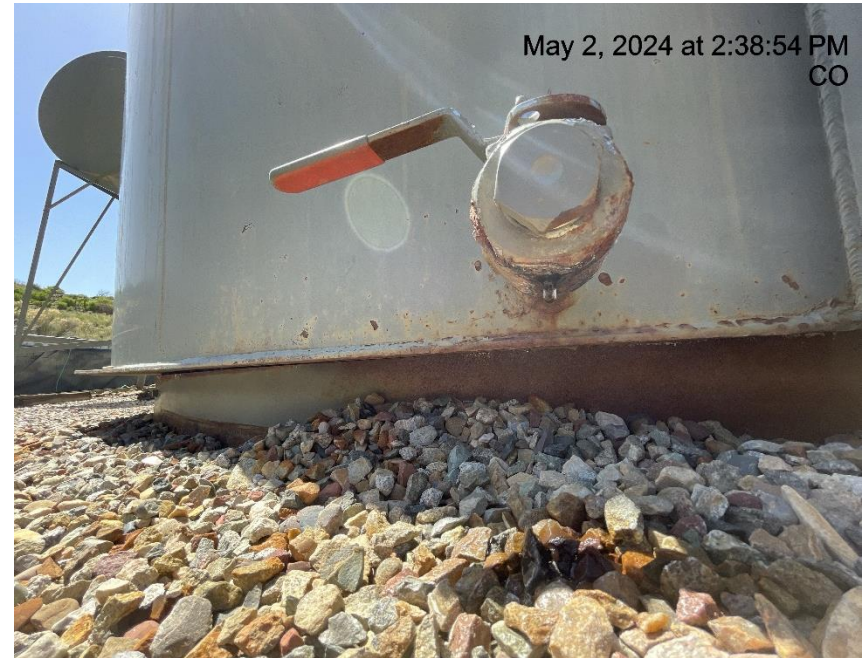
Photo # 5655 Valve on production tank leaking fluid
