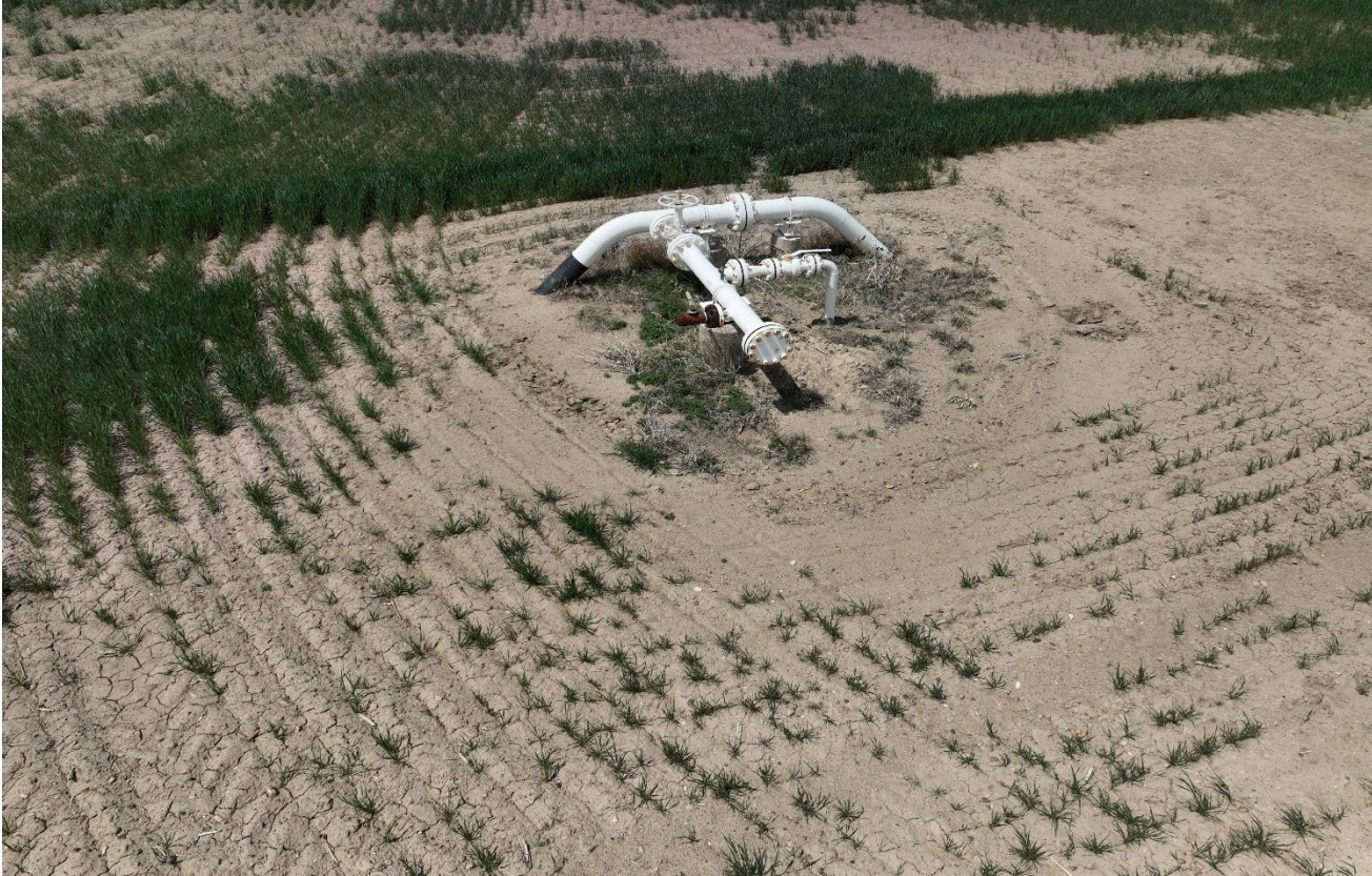
Photo 4. Facing down toward the abandoned wellsite. There are pipe risers and lines that have not been abandoned and removed and are interfering with crop production.
