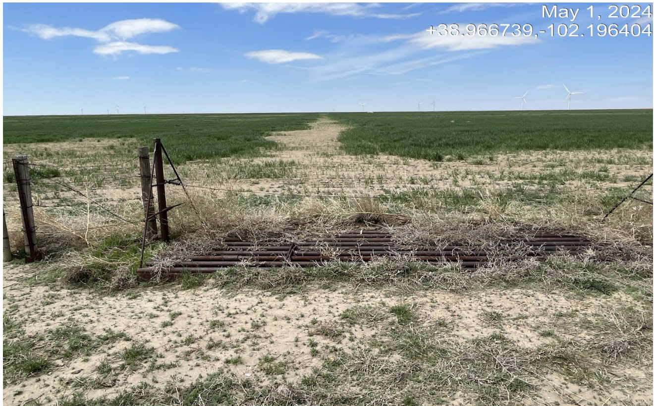
Photo 1. Facing west at the beginning of the access road. The cattleguard has not been removed..
