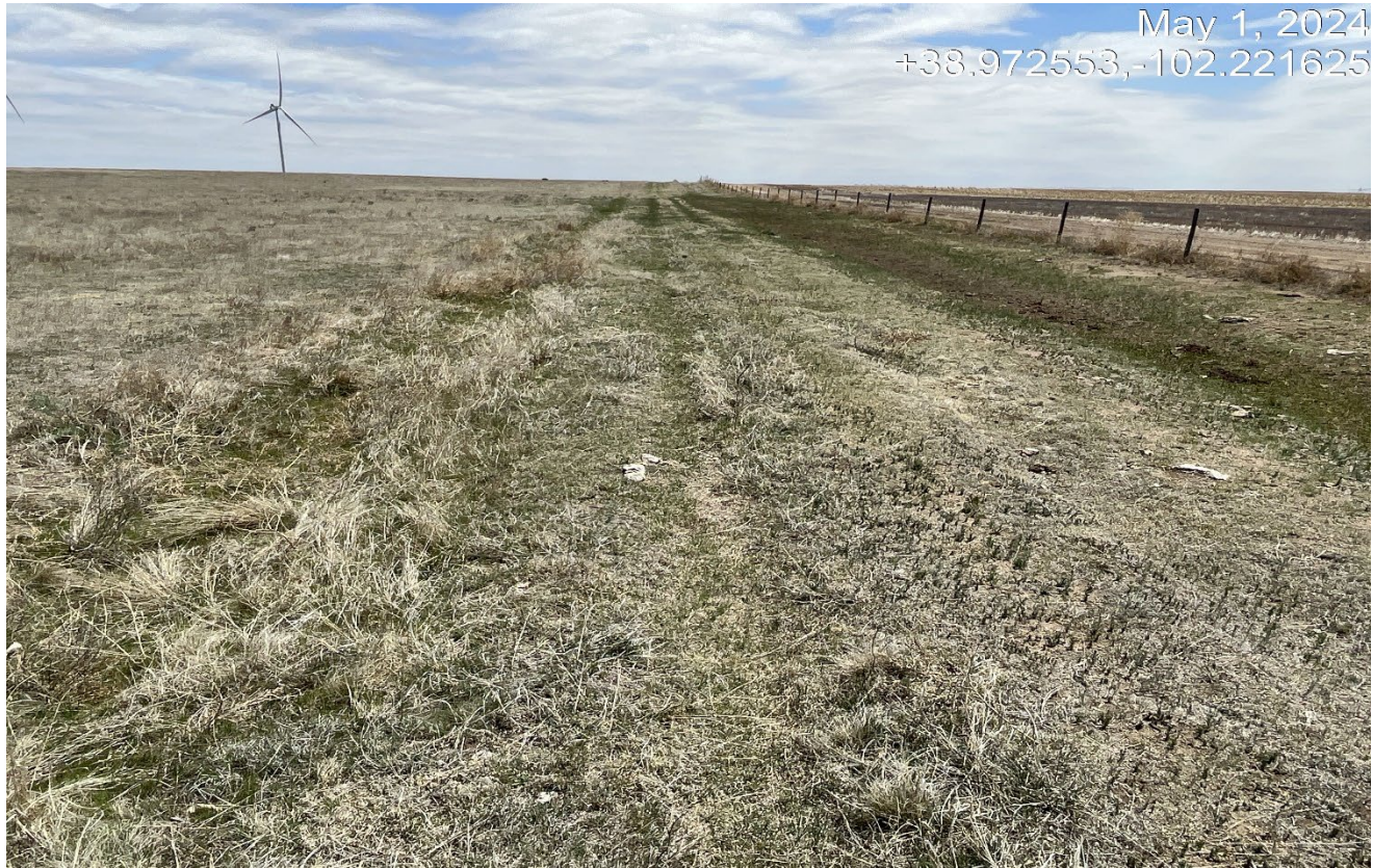
Photo 2. Facing east along the access road. The road was never recontoured. Native vegetation has re-established along the road.
