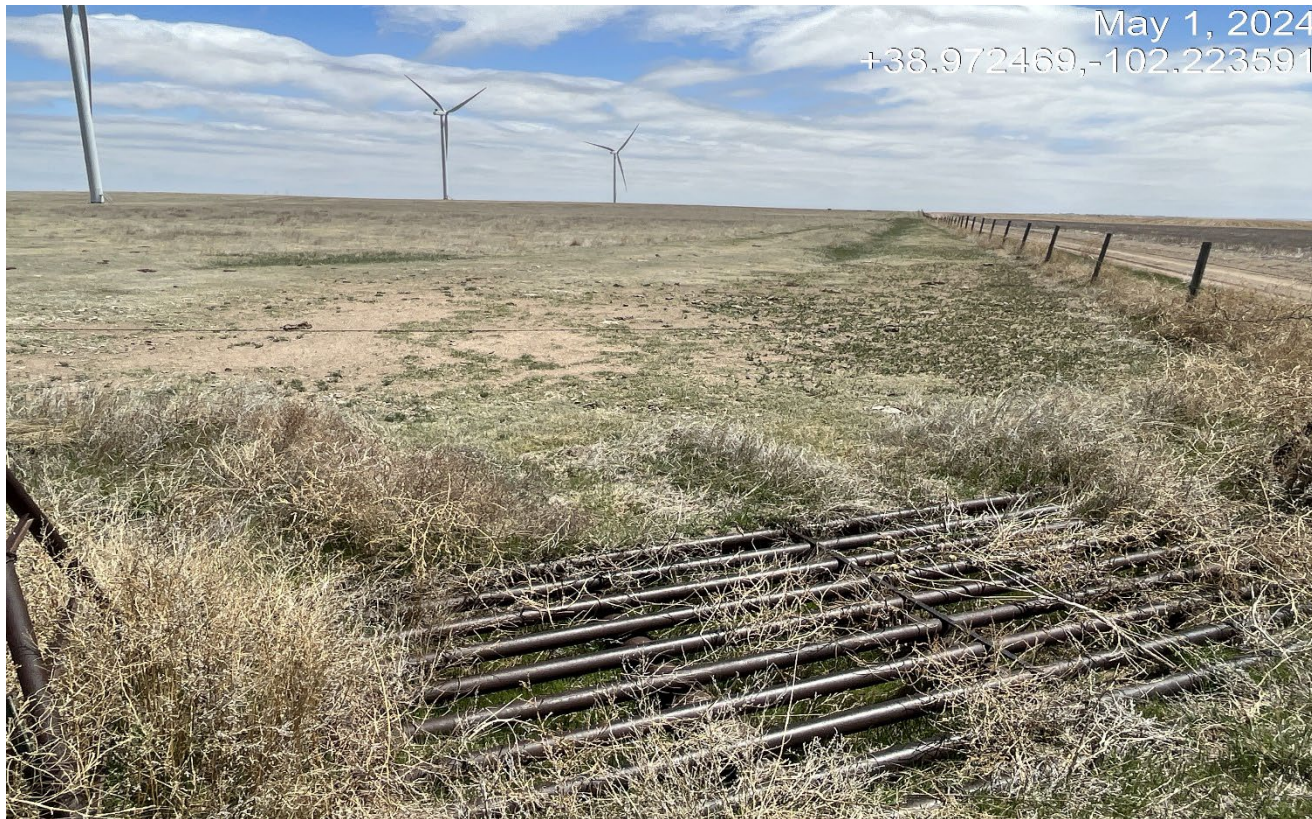
Photo 1. Facing east at the beginning of the access road. The cattleguard has not been removed..
