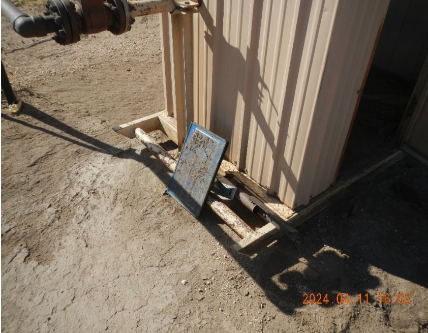
7. Solar Panel was found face down on the ground.
