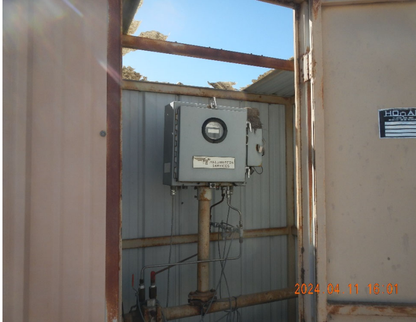
5. Digital gas meter inside meter shed. Roof of meter shed damaged.
