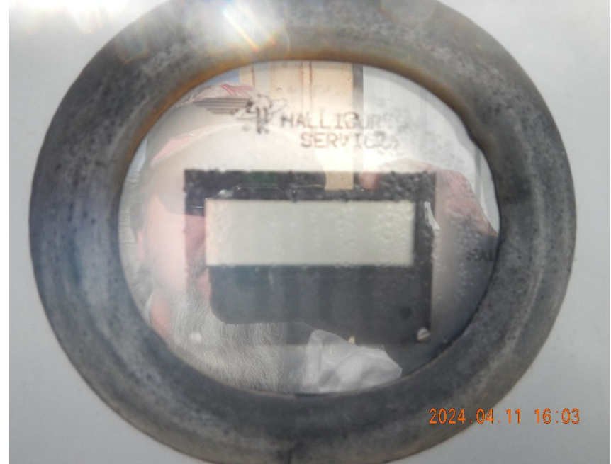
6. Flow meter appears to have no power.
