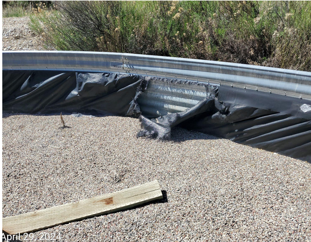
Photo 5: Liner in disrepair at tank battery facility.
