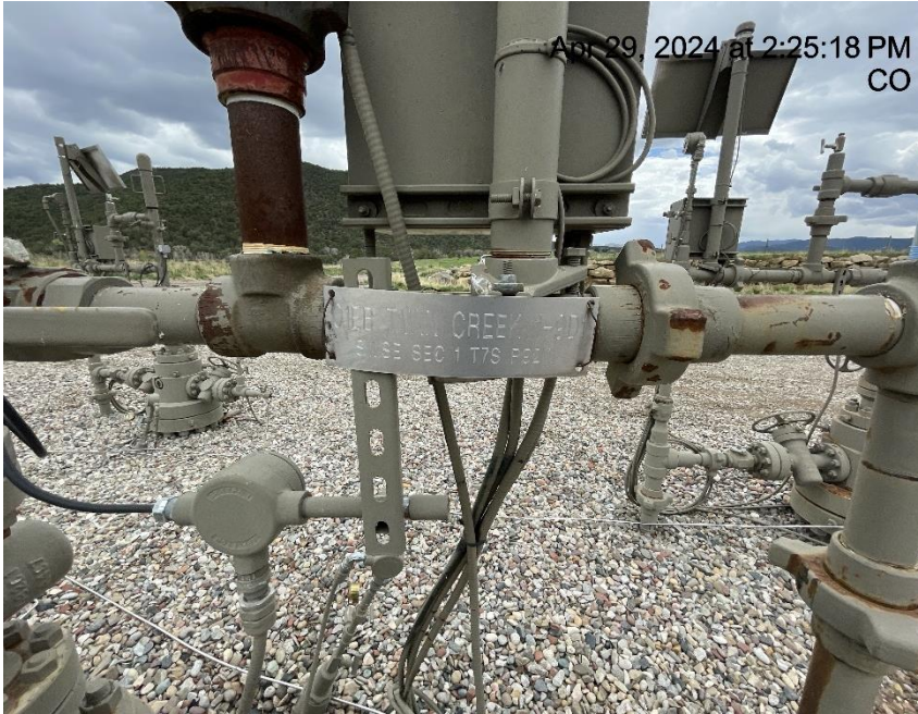
Photo # 5445 Wellhead sign lacks required info
