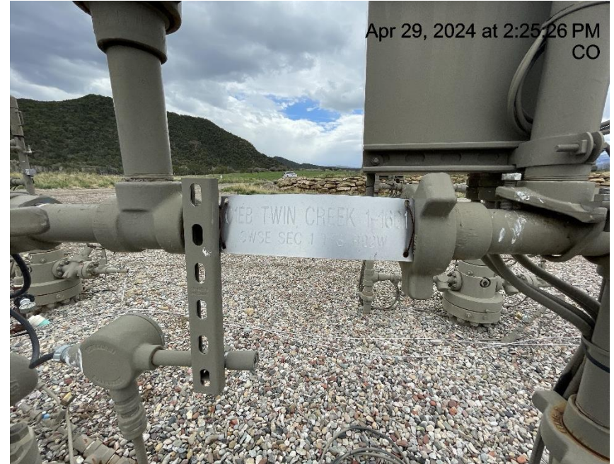
Photo # 5446 Wellhead sign lacks required info
