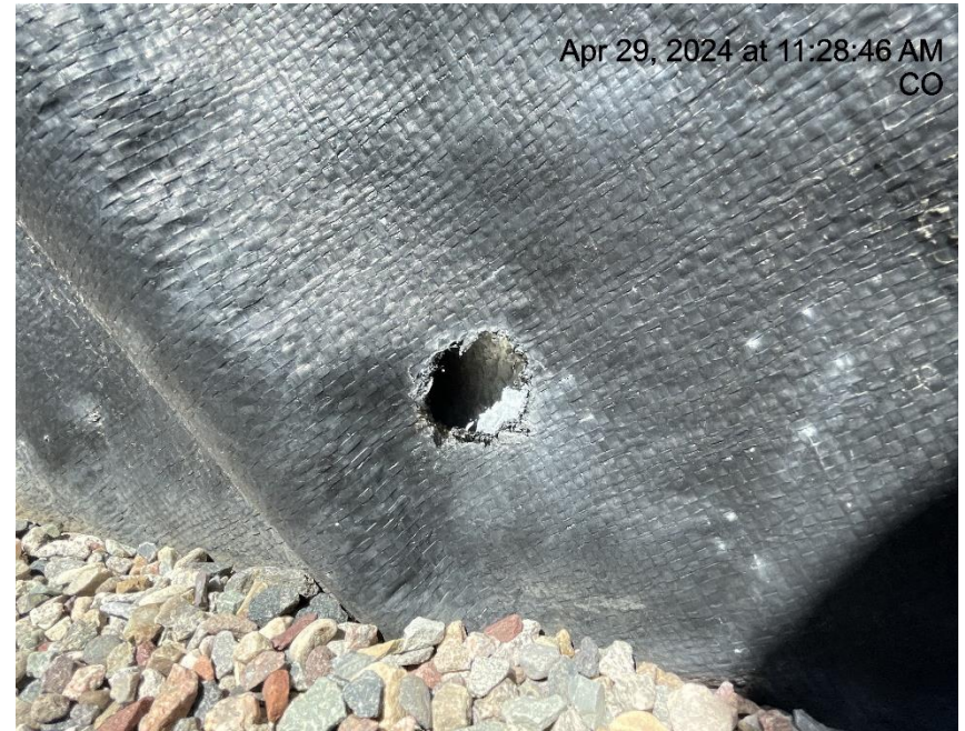
Photo # 5244 Hole in liner/liner needs maintenance
