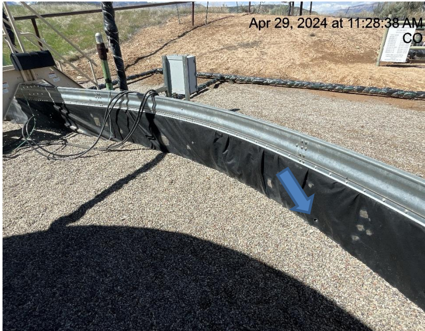
Photo # 5243 Hole in liner/liner needs maintenance
