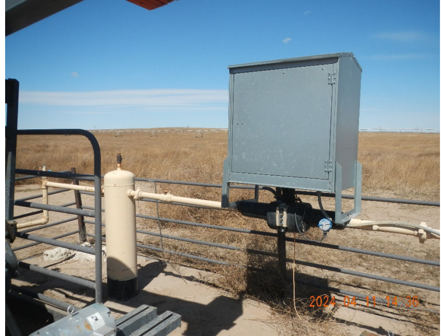
4. Flowline mounted gas meter box.
