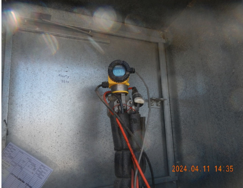
5. Digital gas meter inside meter box.
