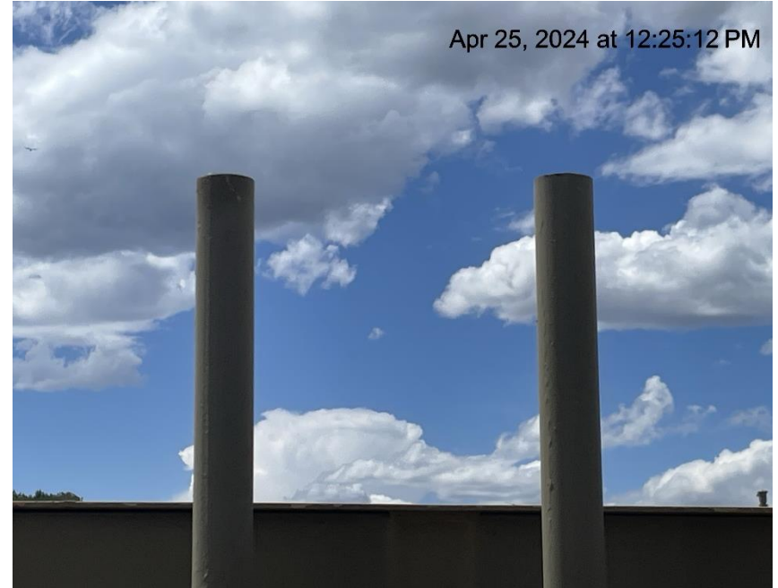
Photo # 5060 PRV & rupture disc vent lines do not comply with CECMC pressure safety device rules
