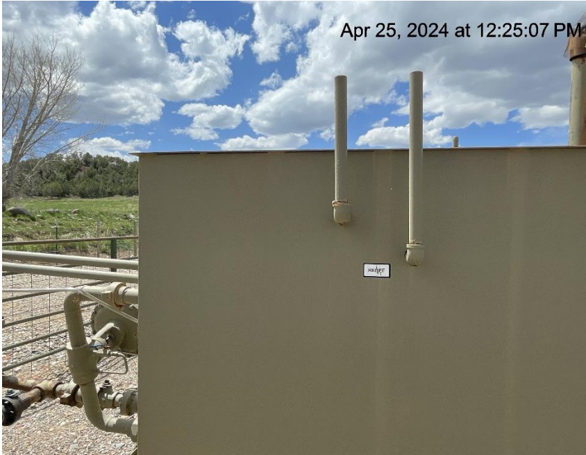
Photo # 5059 PRV & rupture disc vent lines do not comply with CECMC pressure safety device rules
