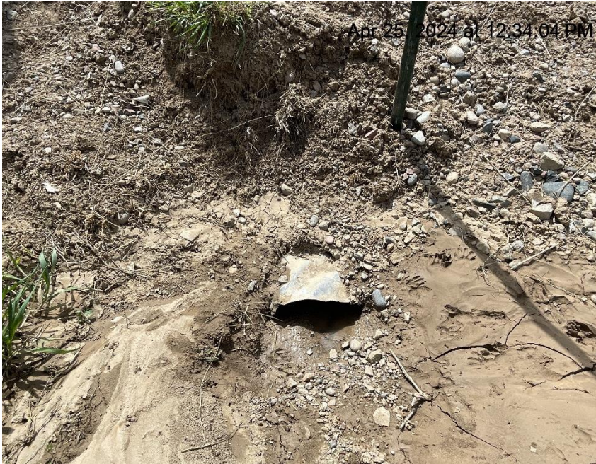
Photo # 5061 Culvert/BMP needs maintenance (on lease road at entrance to location on N/NE side of location)
