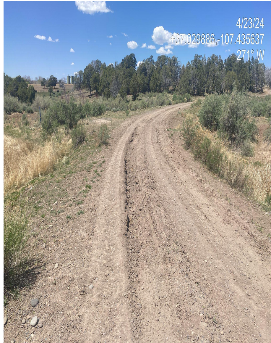
Photo 4. Gully erosion and rutting erosion observed forming along the access road.
