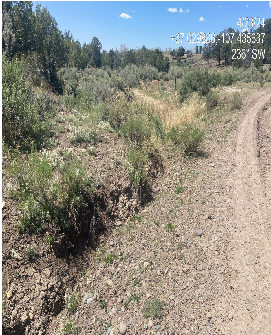
Photo 4. Gully erosion and rutting erosion observed forming along the access road.
