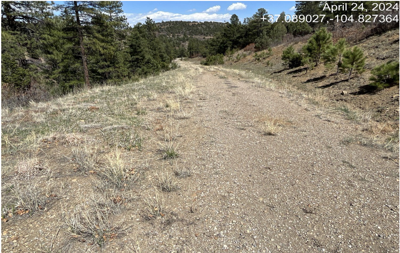
Photo 5. Facing northeast along the road. The remainder of the road is stabilizing well with vegetation.
