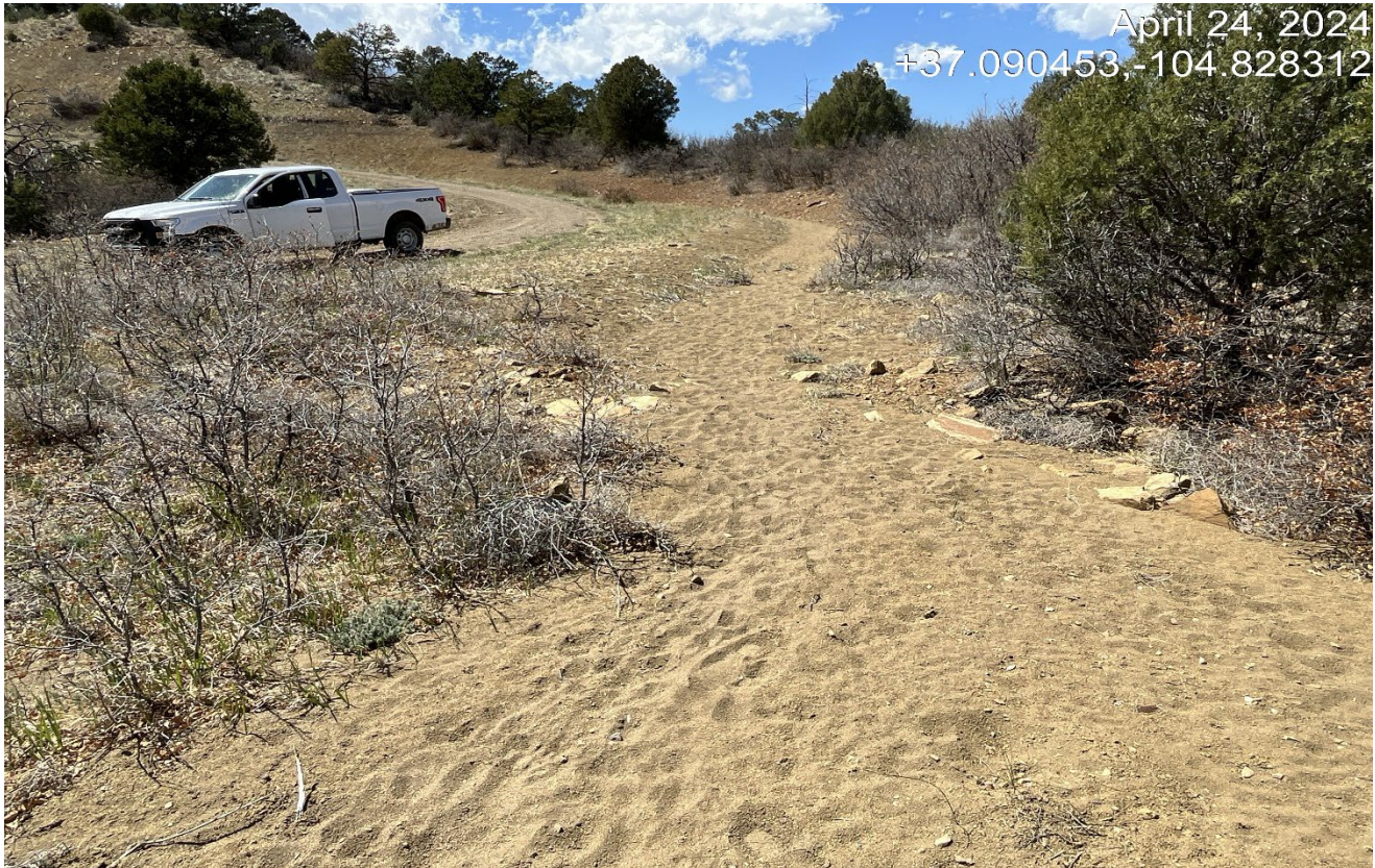
Photo 3. At the switchback of the road there is sediment accumulation that has filled in the rip/tap outlet. This BMP will need to be repaired and additional BMP's should be installed further up the road to prevent erosion.
