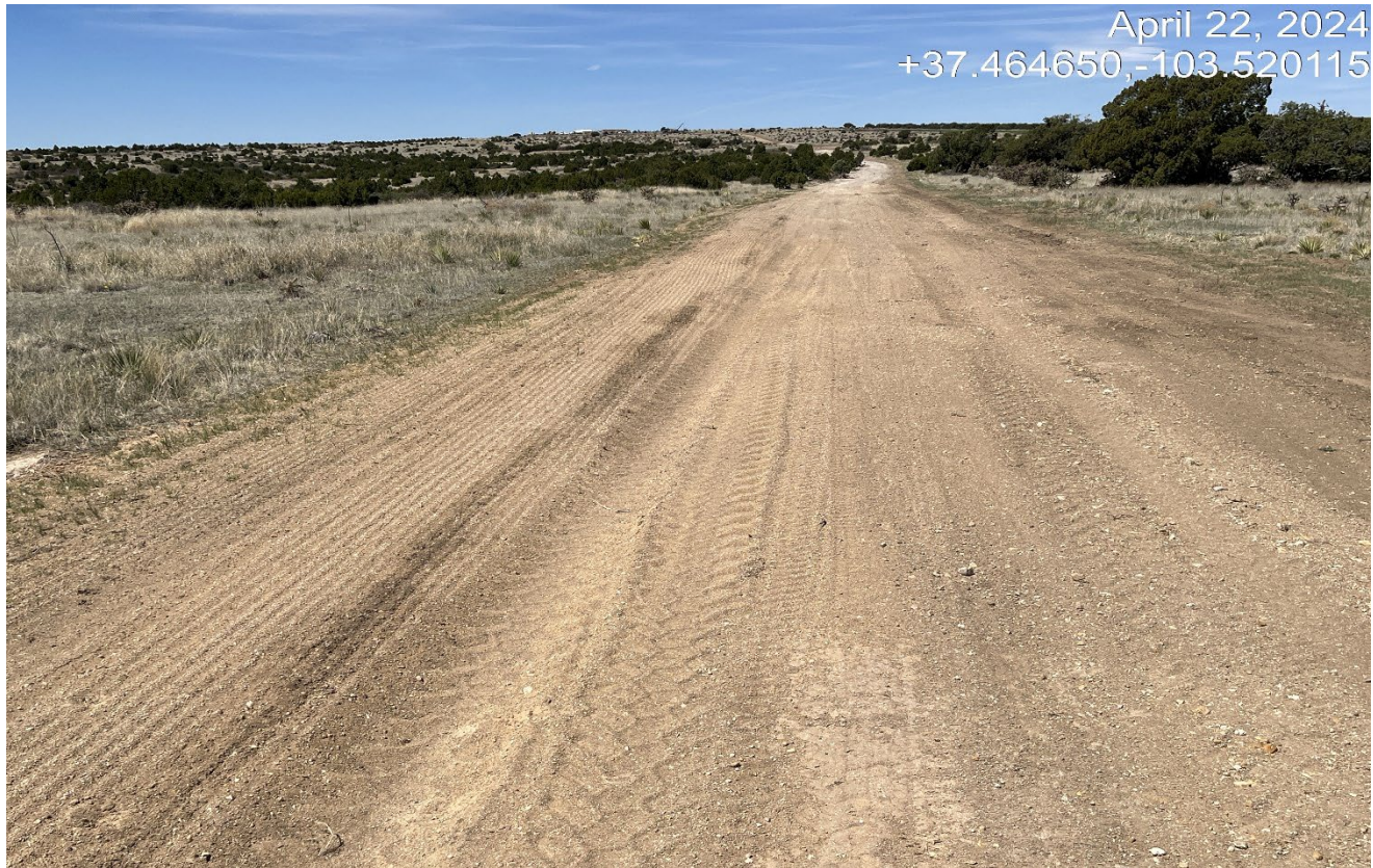
Photo 4. Facing back west toward the flowline disturbance. It appears seeding was performed however loose soils are not stabilized. This area needs to be monitored and additional BMP's may need to be installed.
