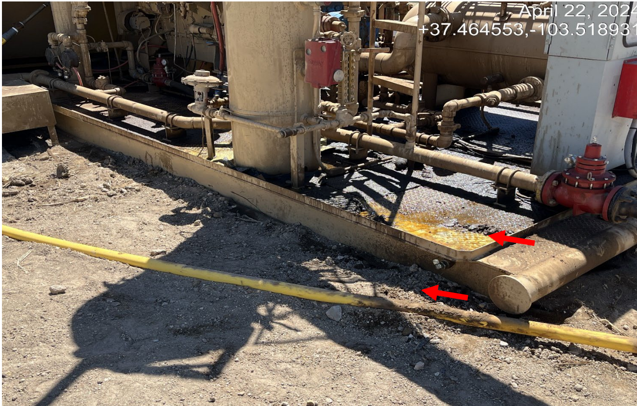
Photo 7. There is oily fluids in the engine skid that has spilled onto the ground. This must be cleaned up.
