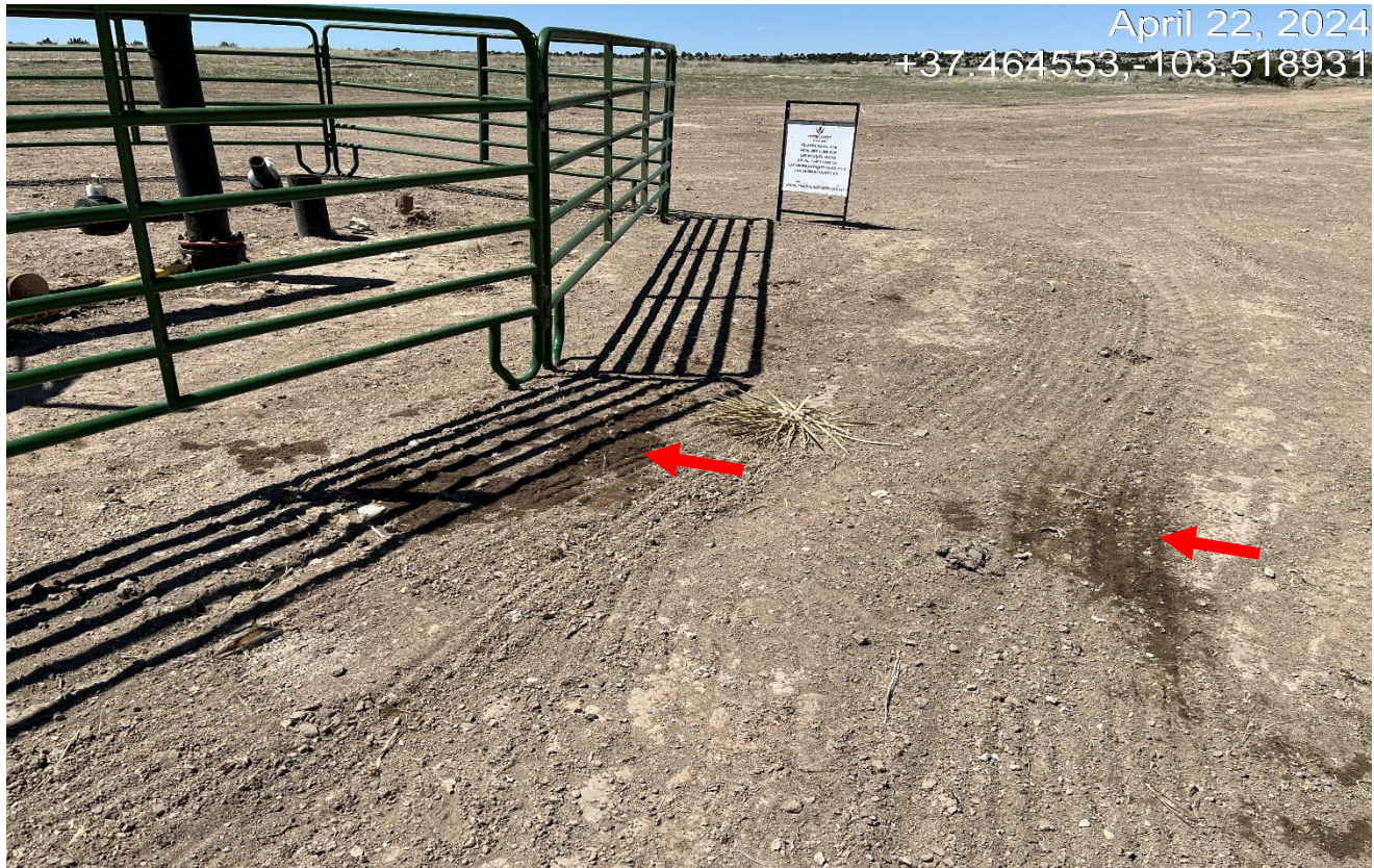
Photo 8. There is stained soil outside fenced area that must be cleaned up.
