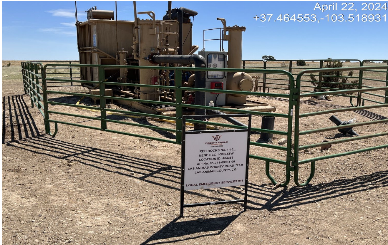
Photo 6. There is compressor engine installed b the wellhead.
