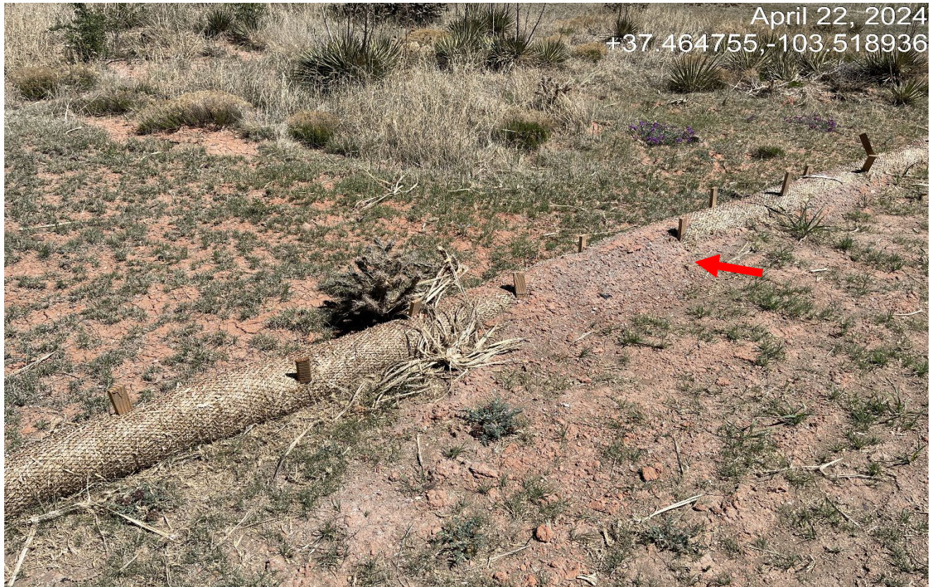
Photo 14. North side of the location are perimeter wattles. There are still red cutting by the wattles.
