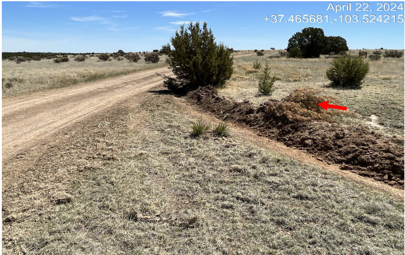
Photo 2. There are cuts installed for stormwater diversion however the loose soil berms need to be stabilized and tree debris must be removed. Previous CA was not completed.
