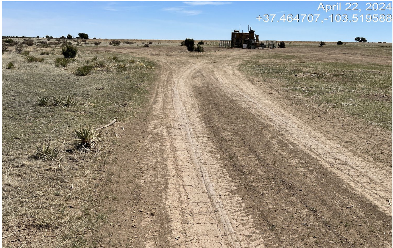
Photo 5. Facing east toward the wellsite. Topsoil was not salvaged along the road and is not very compacted.
