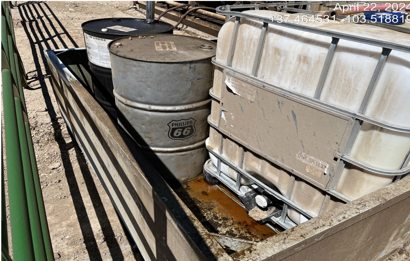
Photo 11. There are fuel containers stored inside of secondary containment but have leaked. This needs to be cleaned up and netting needs to be installed over the top of this area to prevent wildlife entry.
