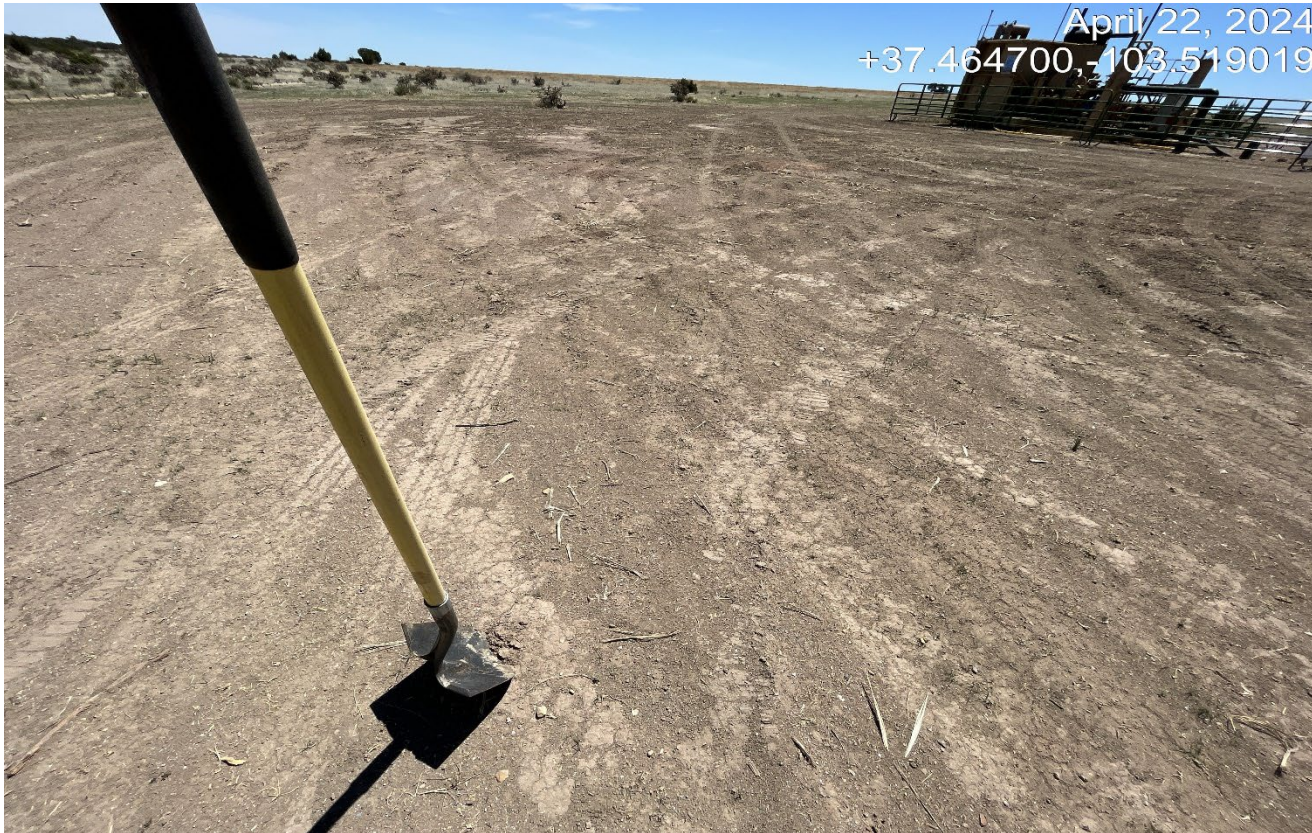
Photo 13. North side of the location facing southwest. There are area where soils are very compacted. Seeding was performed in this area however vegetation will not grow well in compacted soils.
