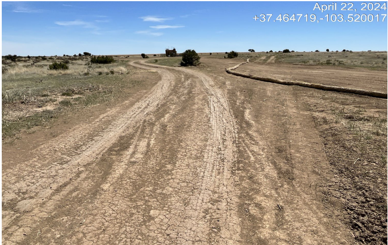
Photo 3. Facing east toward along the access road near the location. Topsoil was not salvaged along the road and is not very compacted.
