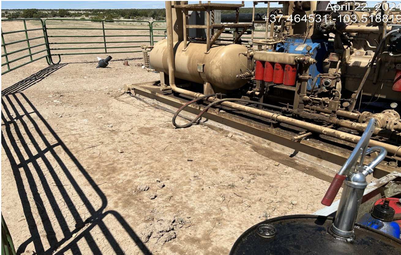
Photo 12. It appears there is more stained soil at around the engine compressor.
